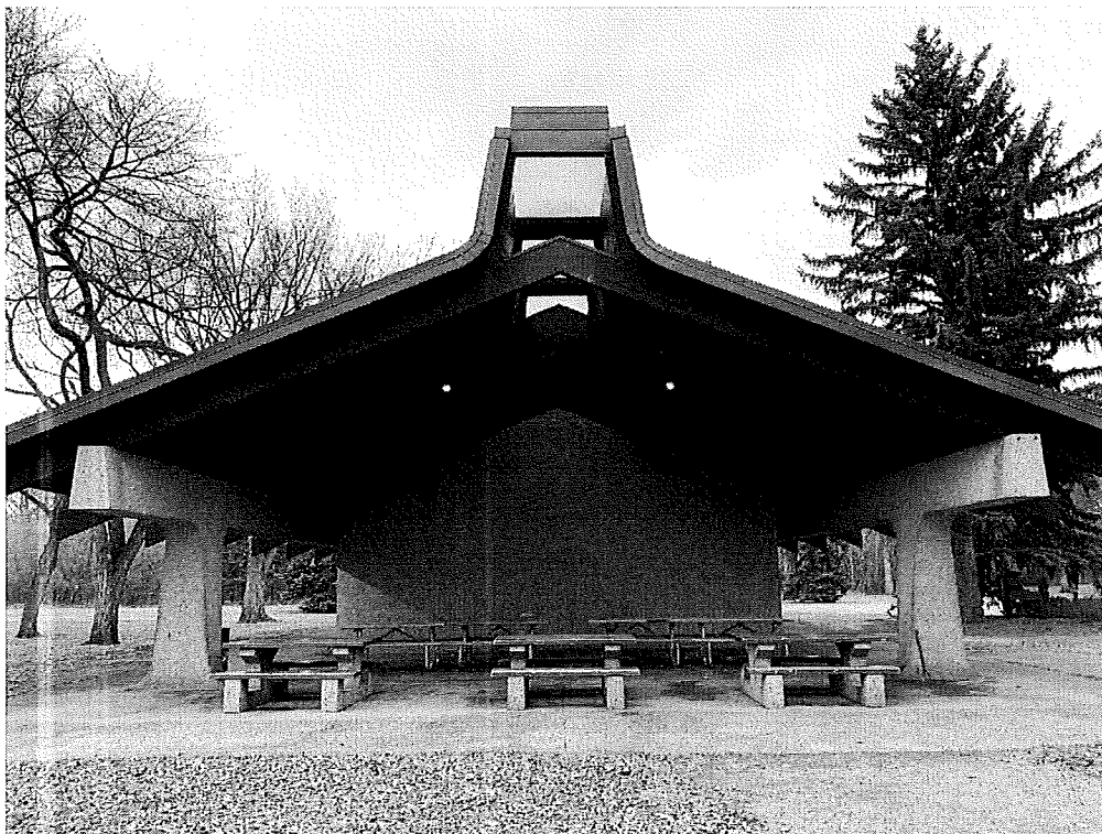
Picnic Shelter #1 south elevation, looking north
