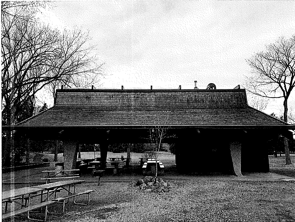
Picnic Shelter #3 east elevation, looking west
