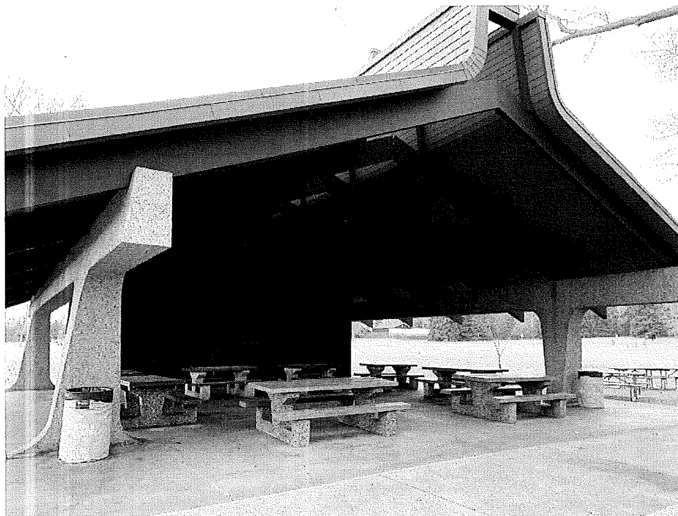
Picnic Shelter #3 south elevation, looking north
