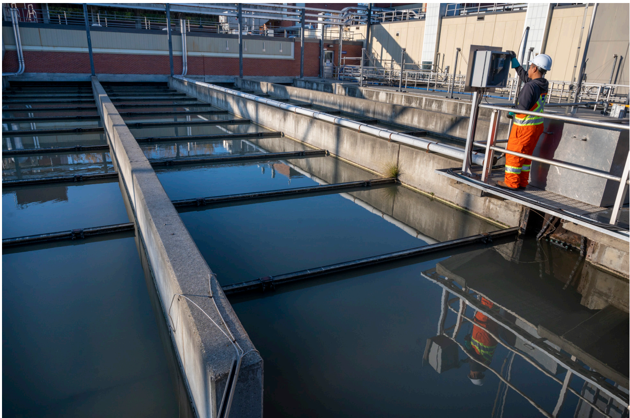
The primary treatment basins at Gold Bar.
