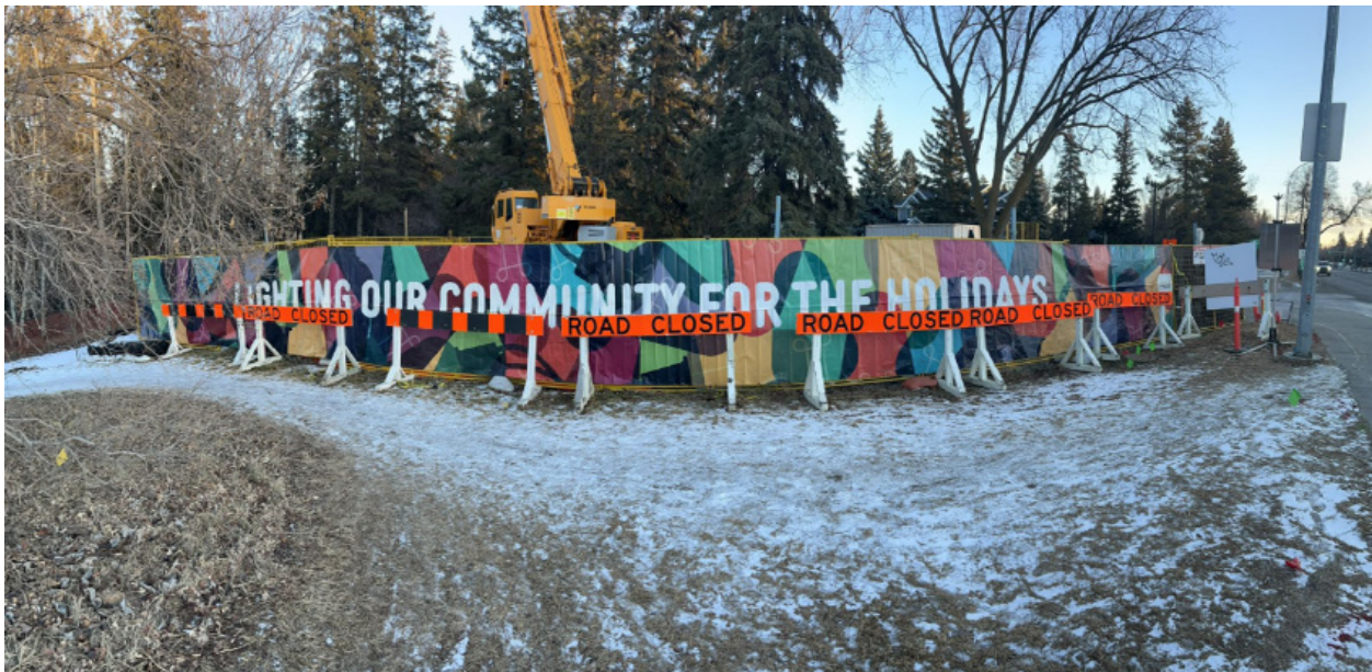
Decorative Art Hoarding installed at 142 Street and Summit Drive as part of the 99 Avenue Trunk Rehabilitation Project
