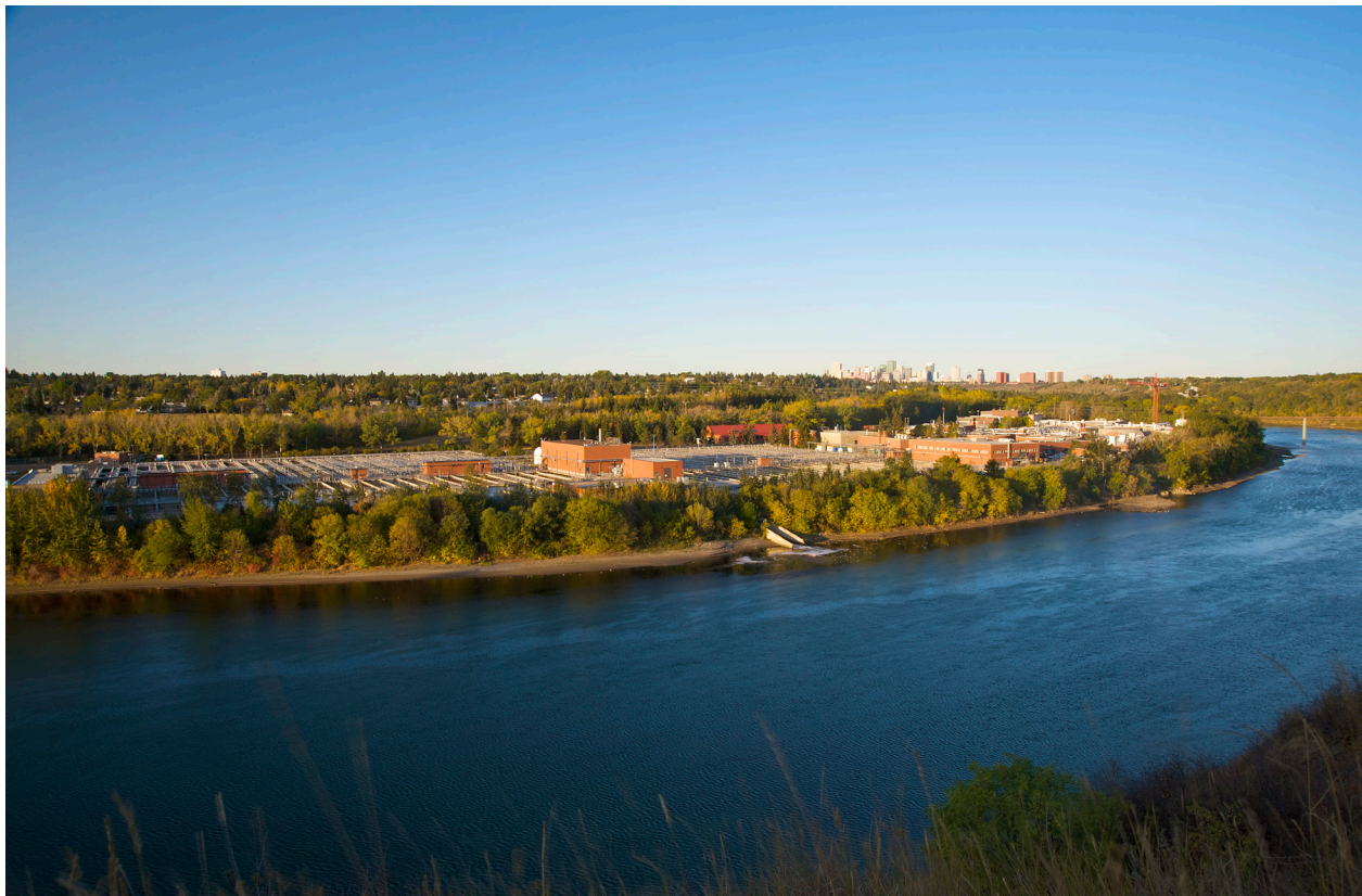
The Gold Bar Wastewater Treatment Plant
