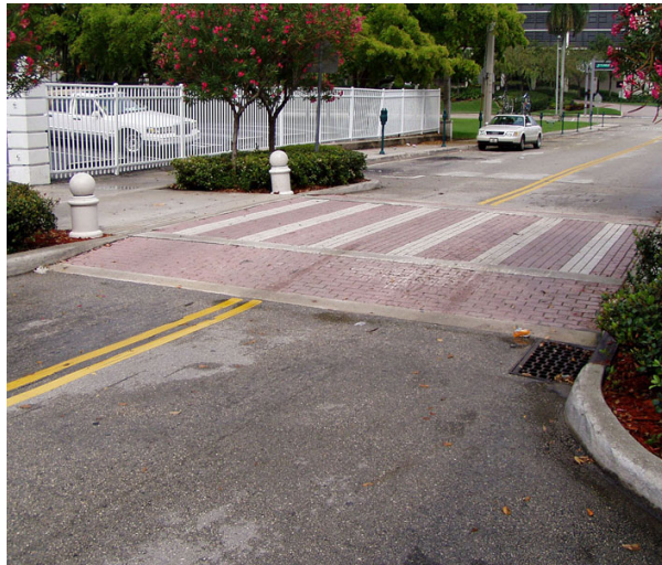
Raised crosswalks such as this one provide traffic calming and uninterrupted grade levels for active mode users, and will be located at crossings along Griesbach Road NW.
