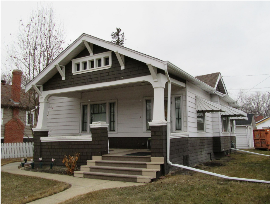
2016, Hunt Residence – south and east elevations (viewed from 109A Avenue NW)
