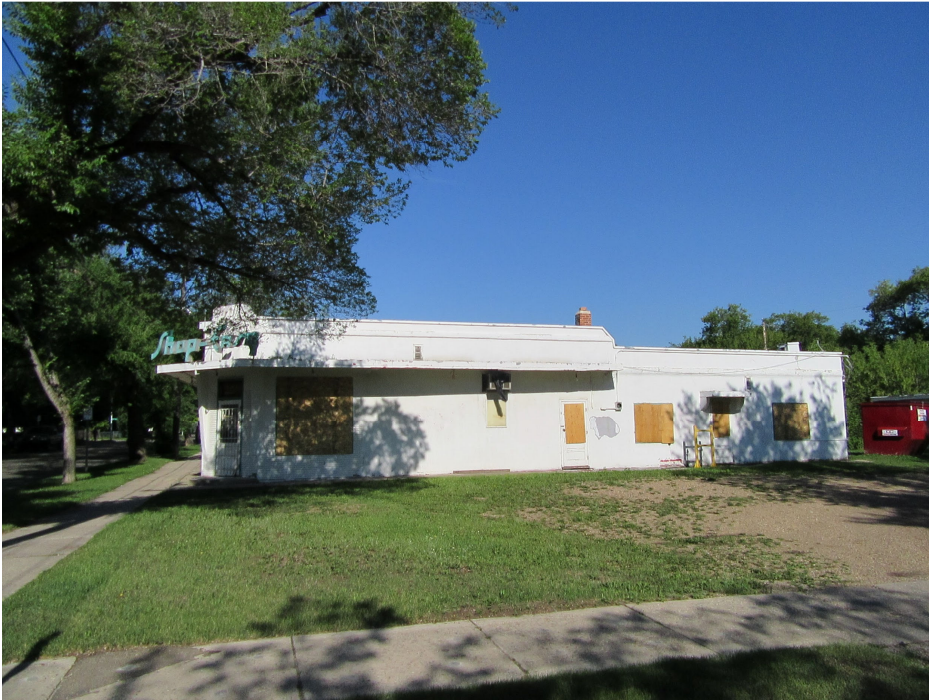
2016, Shop-Easy Grocery – east elevation (viewed from 116 Street NW)
