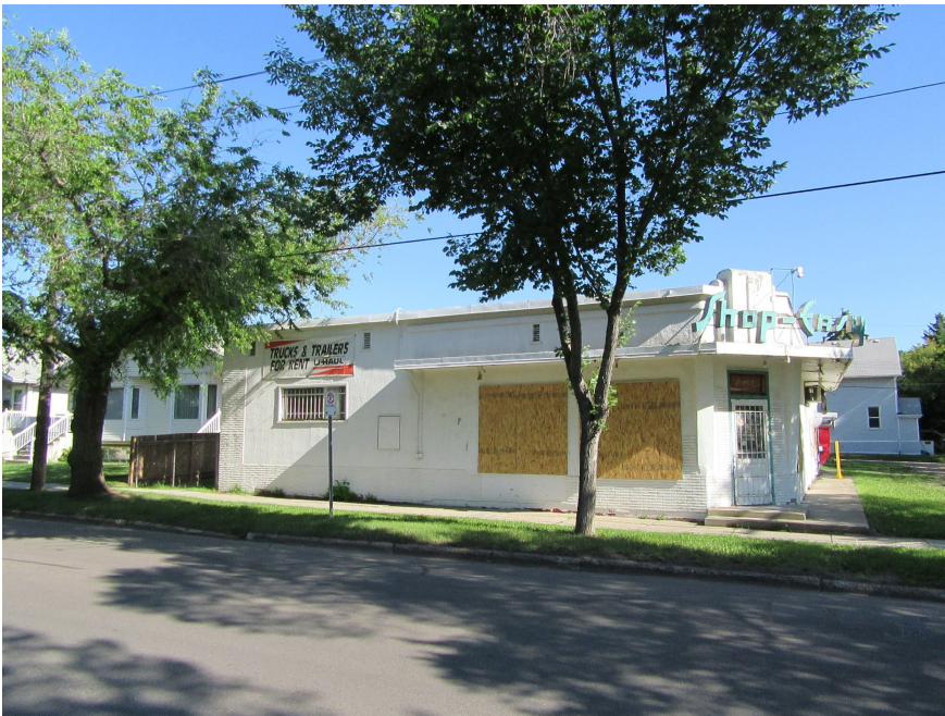
2016, Shop-Easy Grocery – south elevation (viewed from 129 Avenue NW)
