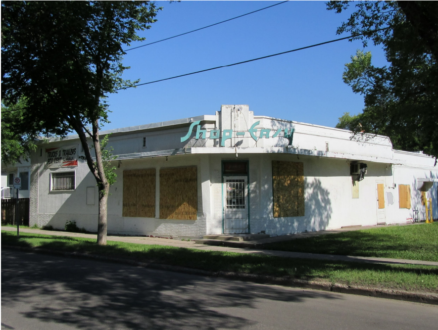
2016, Shop-Easy Grocery – south and east elevations (viewed from 129 Avenue NW)
