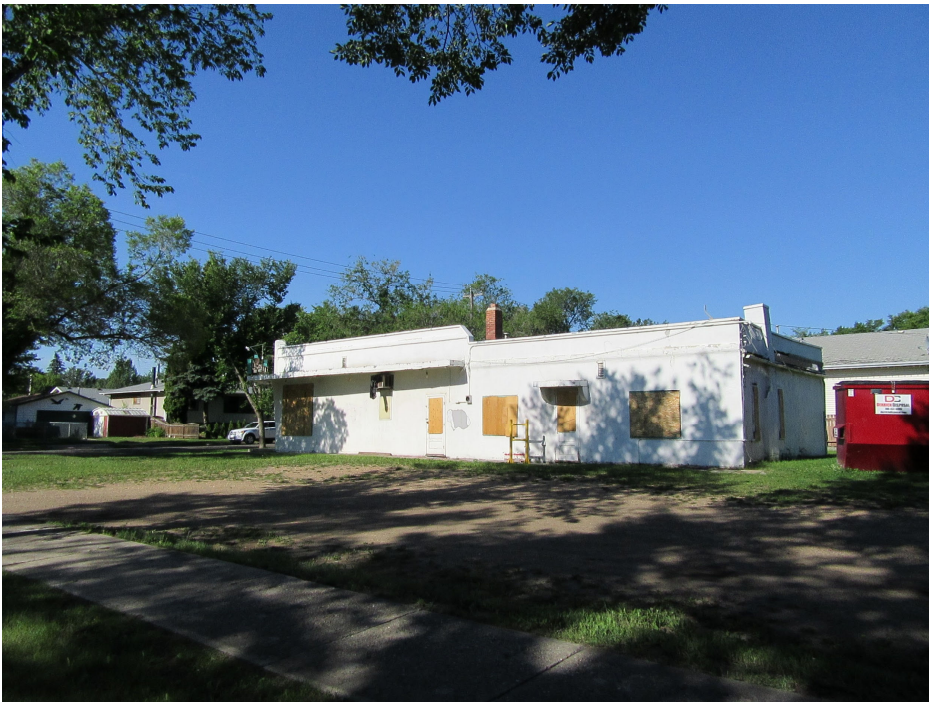
2016, Shop-Easy Grocery – east and north elevations (viewed from 116 Street NW)
