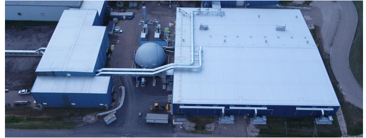
High Solids Anaerobic Digestion Facility
