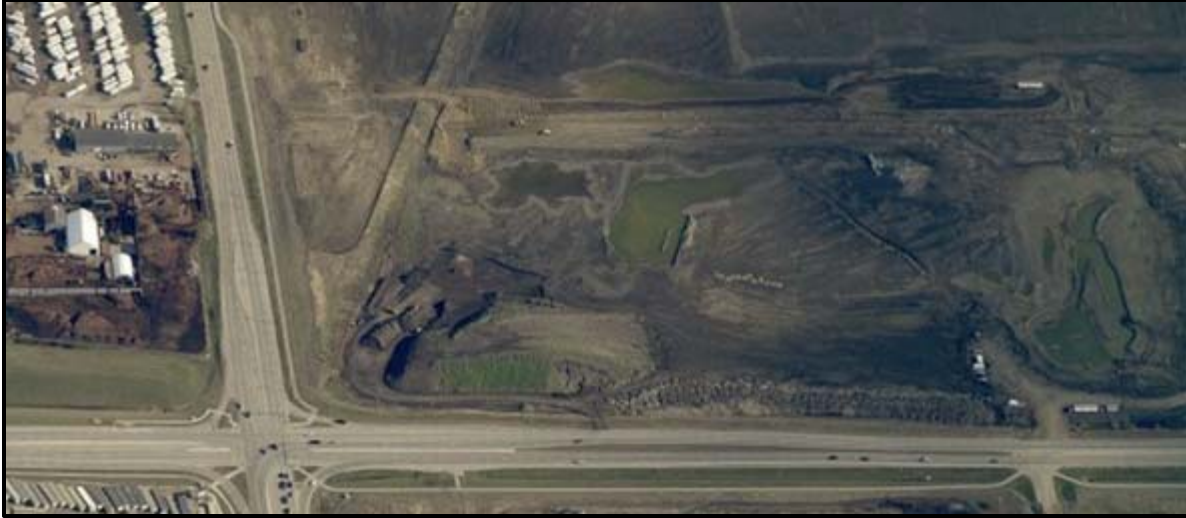
VIEW OF SITE LOOKING NORTH
