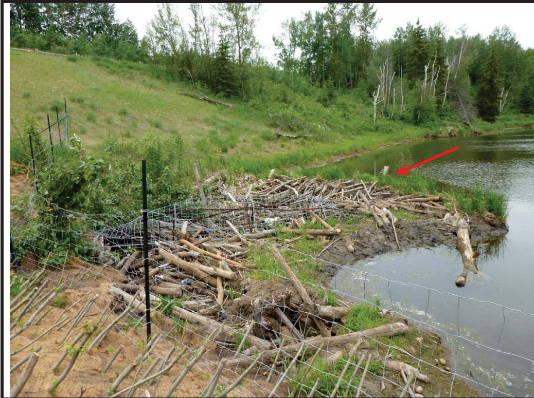
Photo 7: :Looking at upstream end of the culvert Note: Beaver dam, debris catcher and accumulation of debris at upstream end of culvert. Please also note slope of right (south) bank slope.
