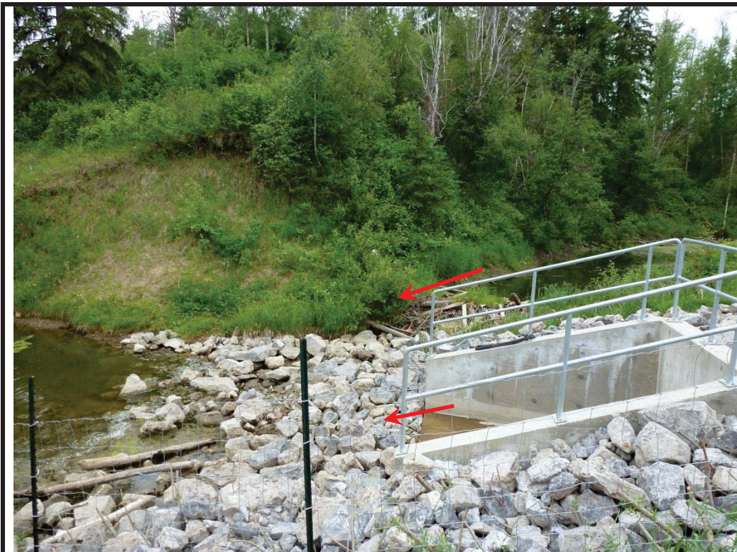
Photo 8: Looking at outfall and its bank protection north of upstream end of culvert
