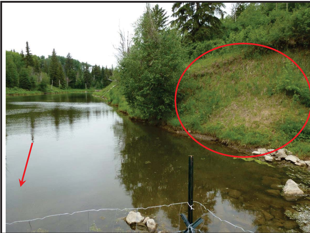
Photo 5: Looking at outfall and its bank protection north of upstream end of culvert Note: Left (north) bank sign of old slumping
