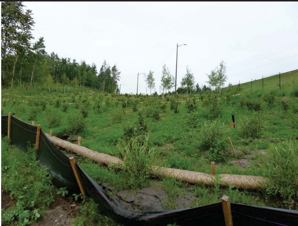
Photo 10: Looking at erosion control measures along upstream (west) side slope
