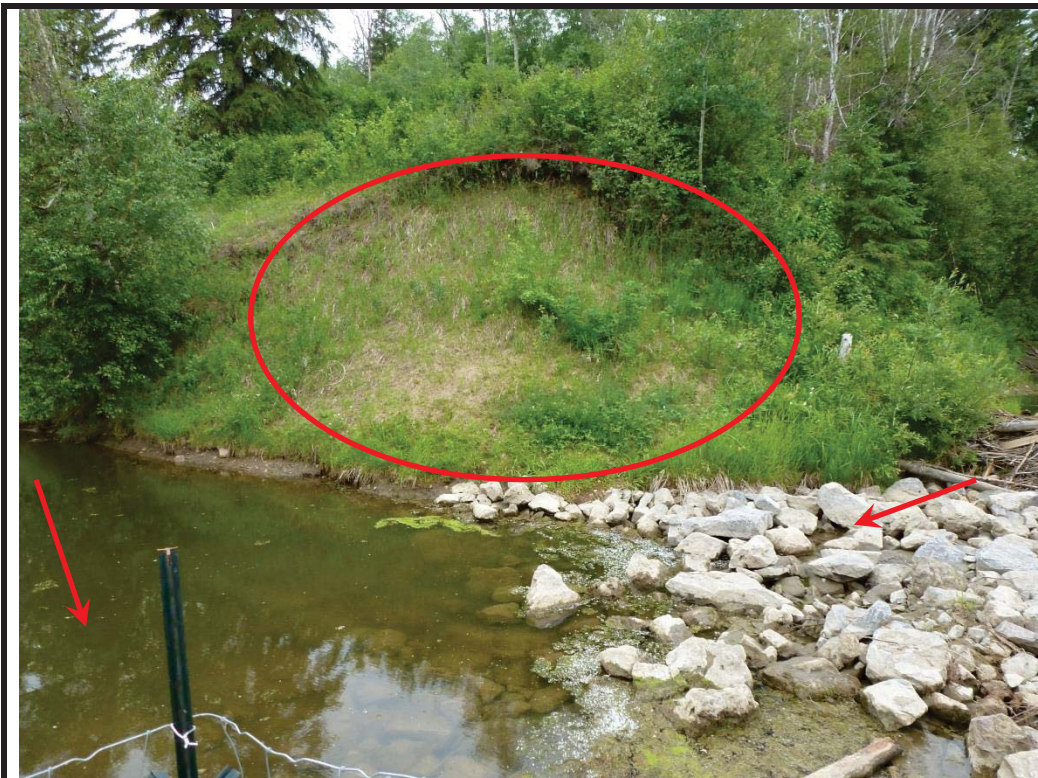
Photo 4: Looking at outfall and its bank protection north of upstream end of culvert Note: Left bank sign of old slumping
