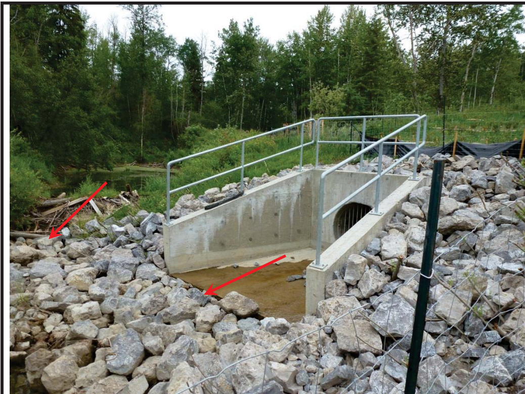
Photo 6: Looking at outfall and its bank protection north of upstream end of culvert Note: Beaver dam at mouth of tributary joining Wedgewood creek
