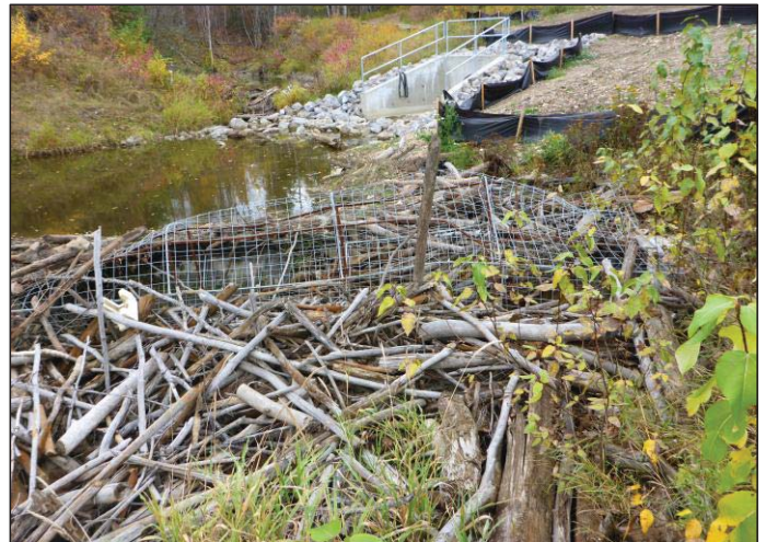
Photo 6: Beaver dam on a culvert upstream of the road crossing creating a temporary fish barrier and flooding areas upstream.
