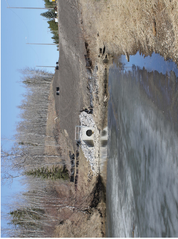
Photo 7: Storm outfall and beaver dam on west sideslope of 199th Street.
