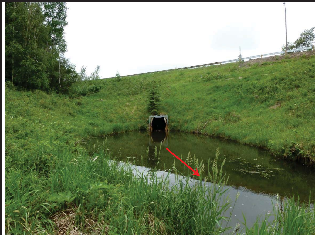
Photo 28: Looking upstream at downstream end of existing culvert Note: scour hole and water ponding (due to beaver dam)
