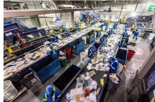
Materials Recovery Facility Renewal
