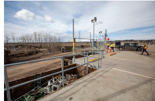
Residential Transfer Station upgrades
