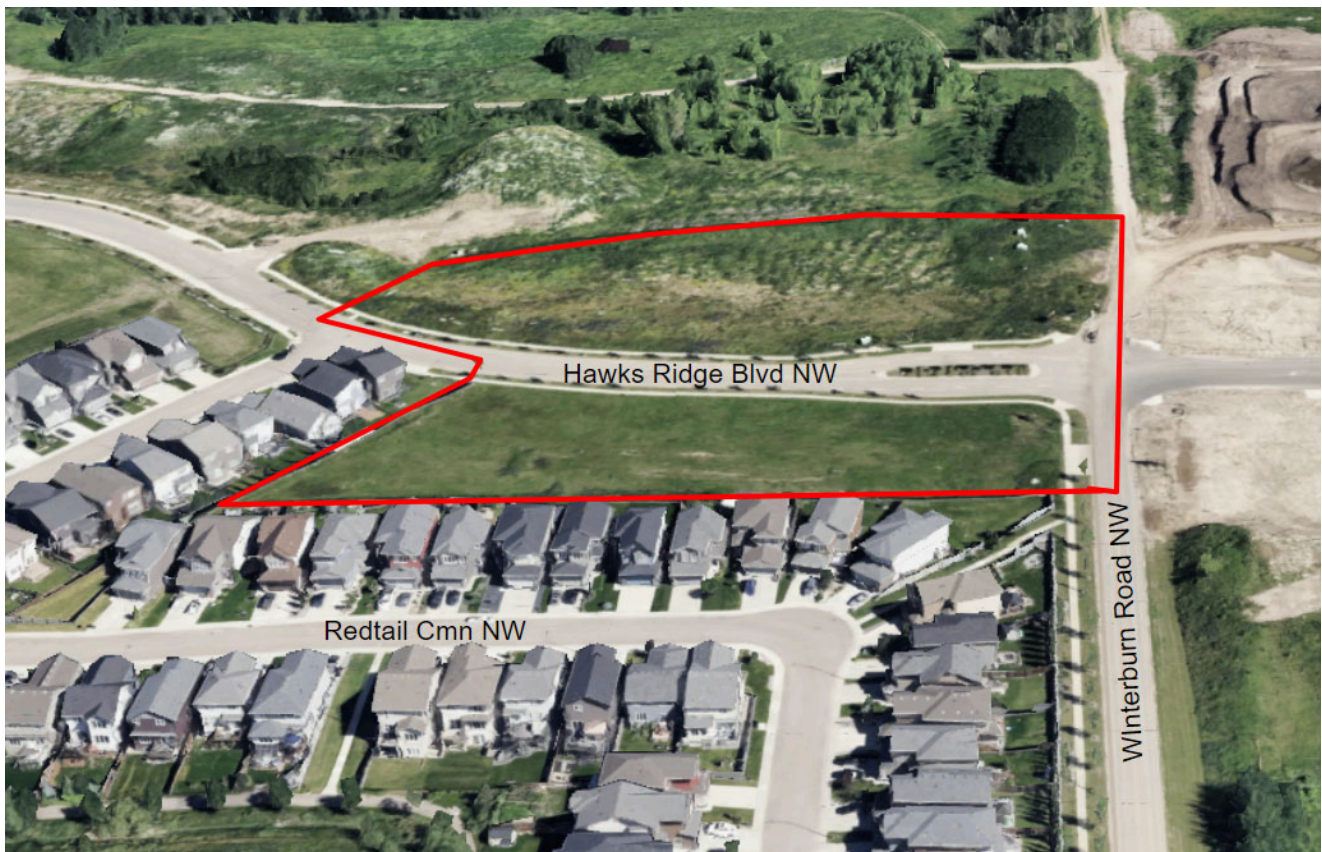
View of site looking north
