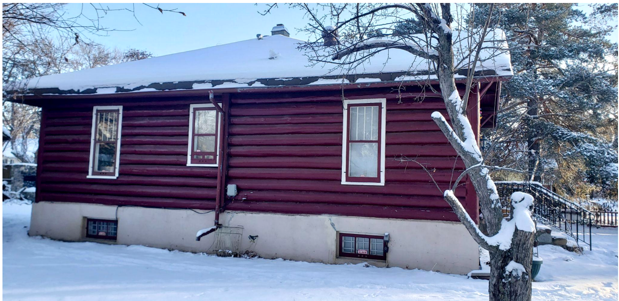
View of north elevation, looking south
