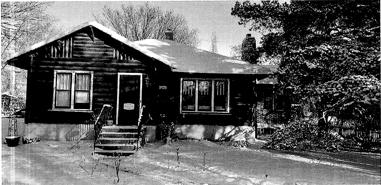
View of west (front) elevation, looking east from 68 Street NW
