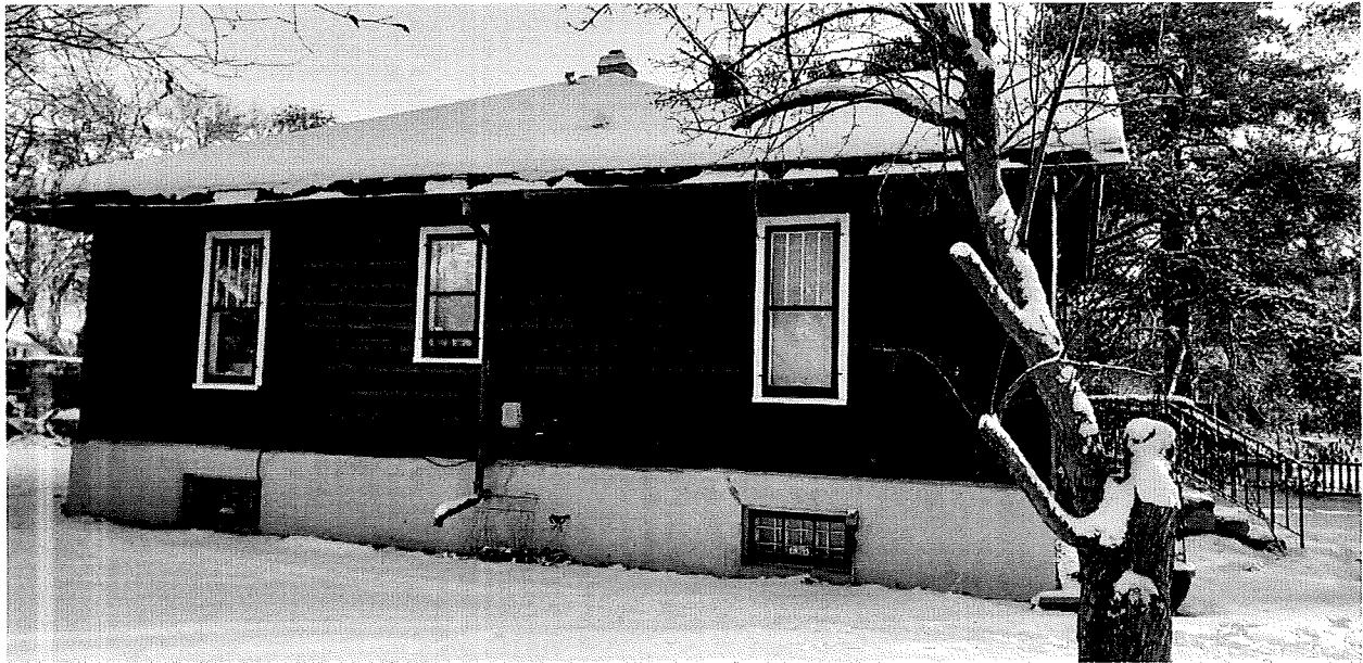
View of north elevation, looking south
