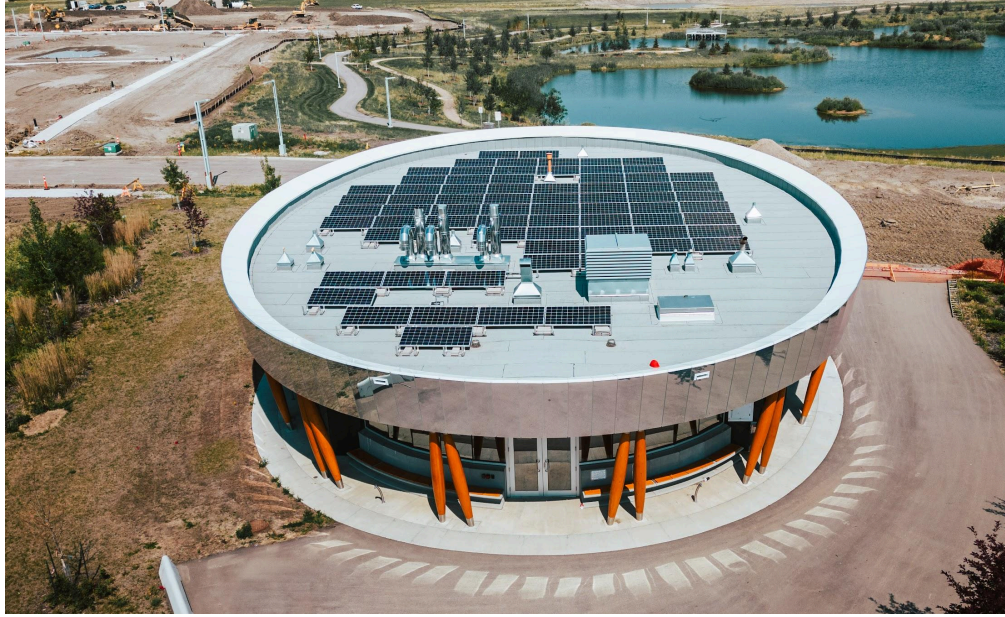
Solar panels installed on the Energy Centre's roof – along with a high-performance building envelope to reduce energy loss to the outdoors, ultra-high performance windows and LED lighting – reflect the sustainability ideals of the community.
