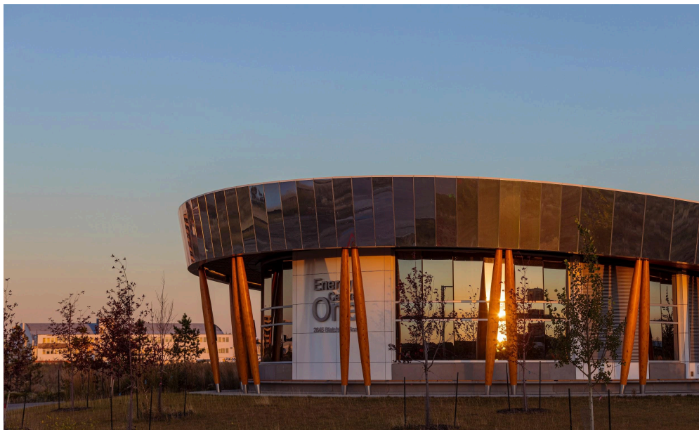
Energy Centre One harnesses earth's geothermal renewable energy for use in the community's District Energy Sharing System.
