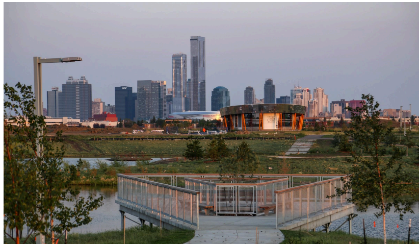
The community's first geexchange field is located underneath the stormwater pond in the community.
