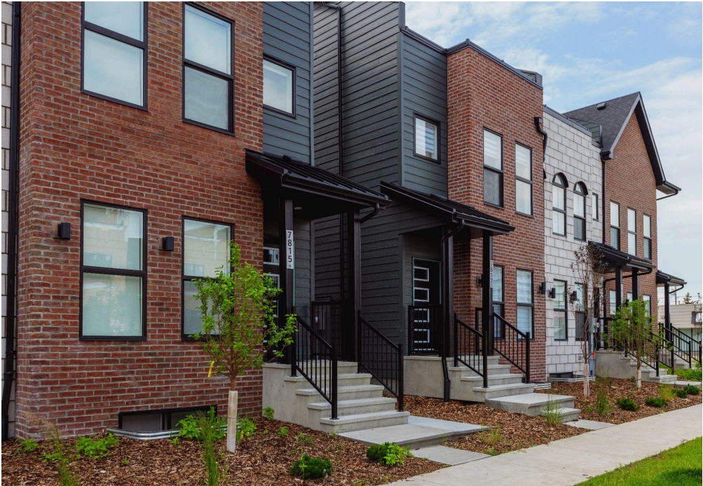
Homes in the community are receiving renewable heating, cooling and hot water services from Blatchford Renewable Energy.
