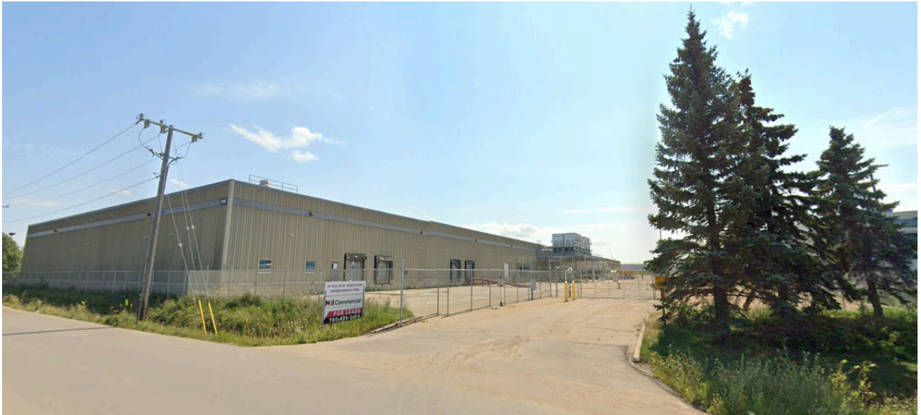
View of the site from 84 Avenue NW
