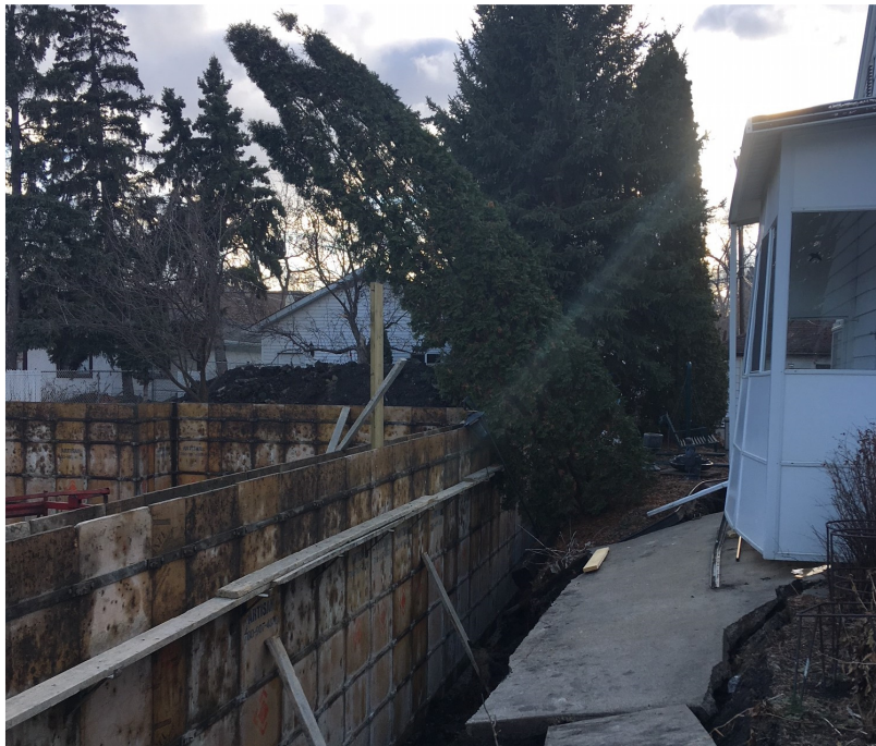
Movement retaining material toward excavation
