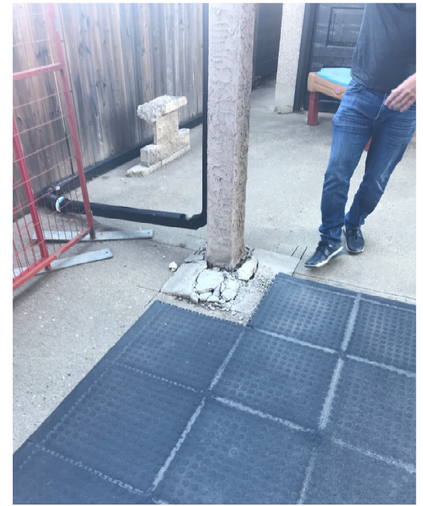
Settlement piles for addition
