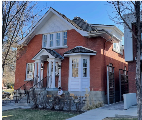
Stopgap Coffee (Oliver) Building Floor Area: ~160 m 2 * *Stopgap Coffee only occupies a portion of the building
