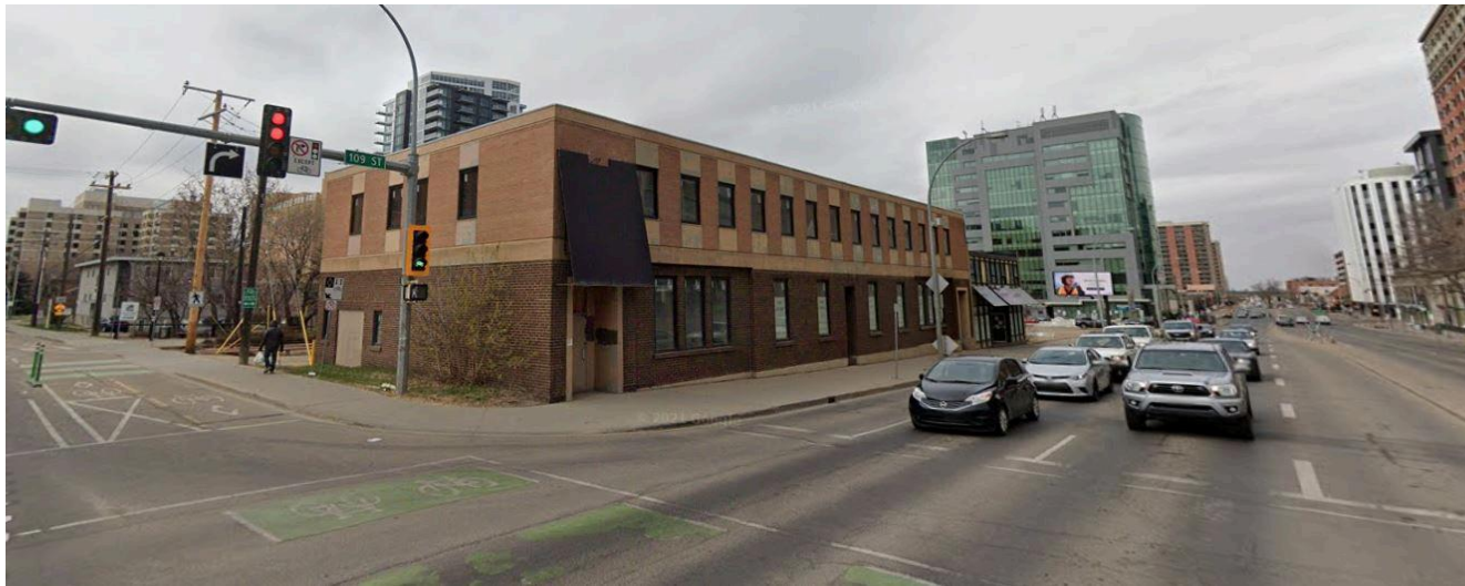
View of a two-storey building from 100 Avenue and 109 Street, facing northwest
