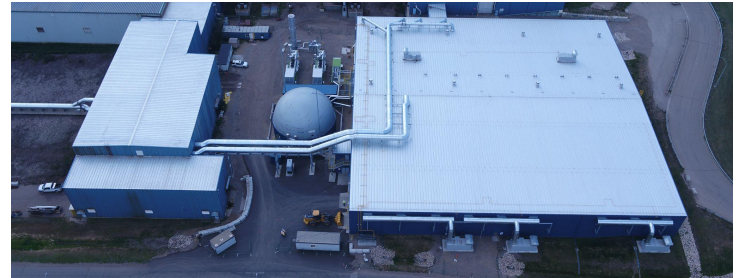
High Solids Anaerobic Digestion Facility
