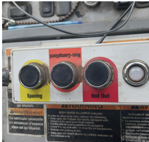
Figure 3: Three-Button System In Truck Cab
