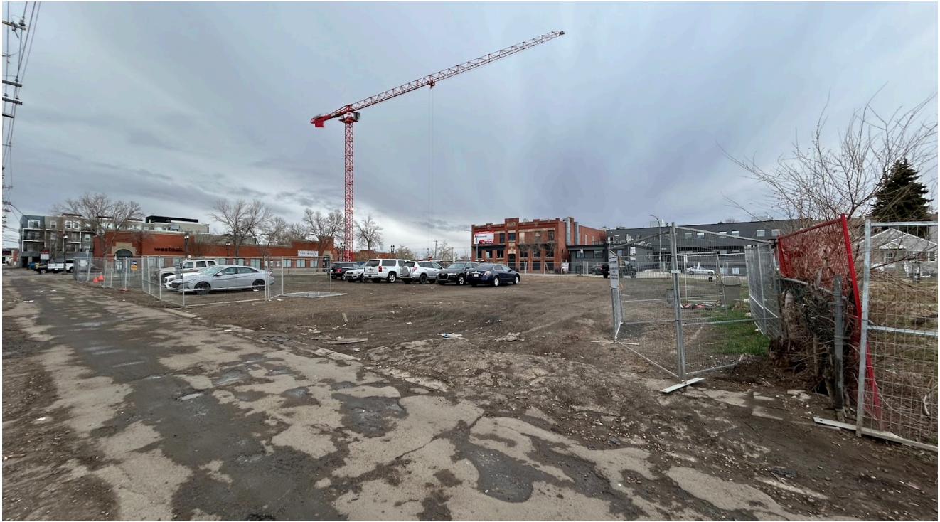
View of site looking southeast from the rear alley
