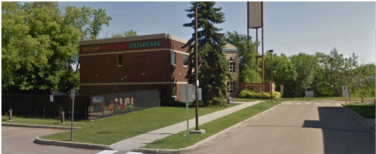
View of site looking northeast
