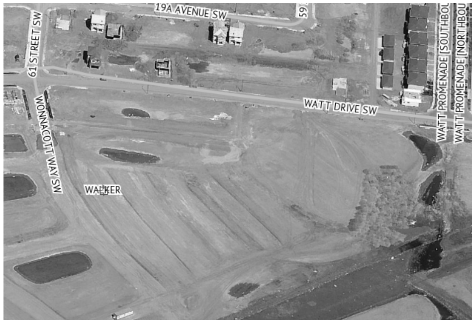
Pictometry View of site looking north
