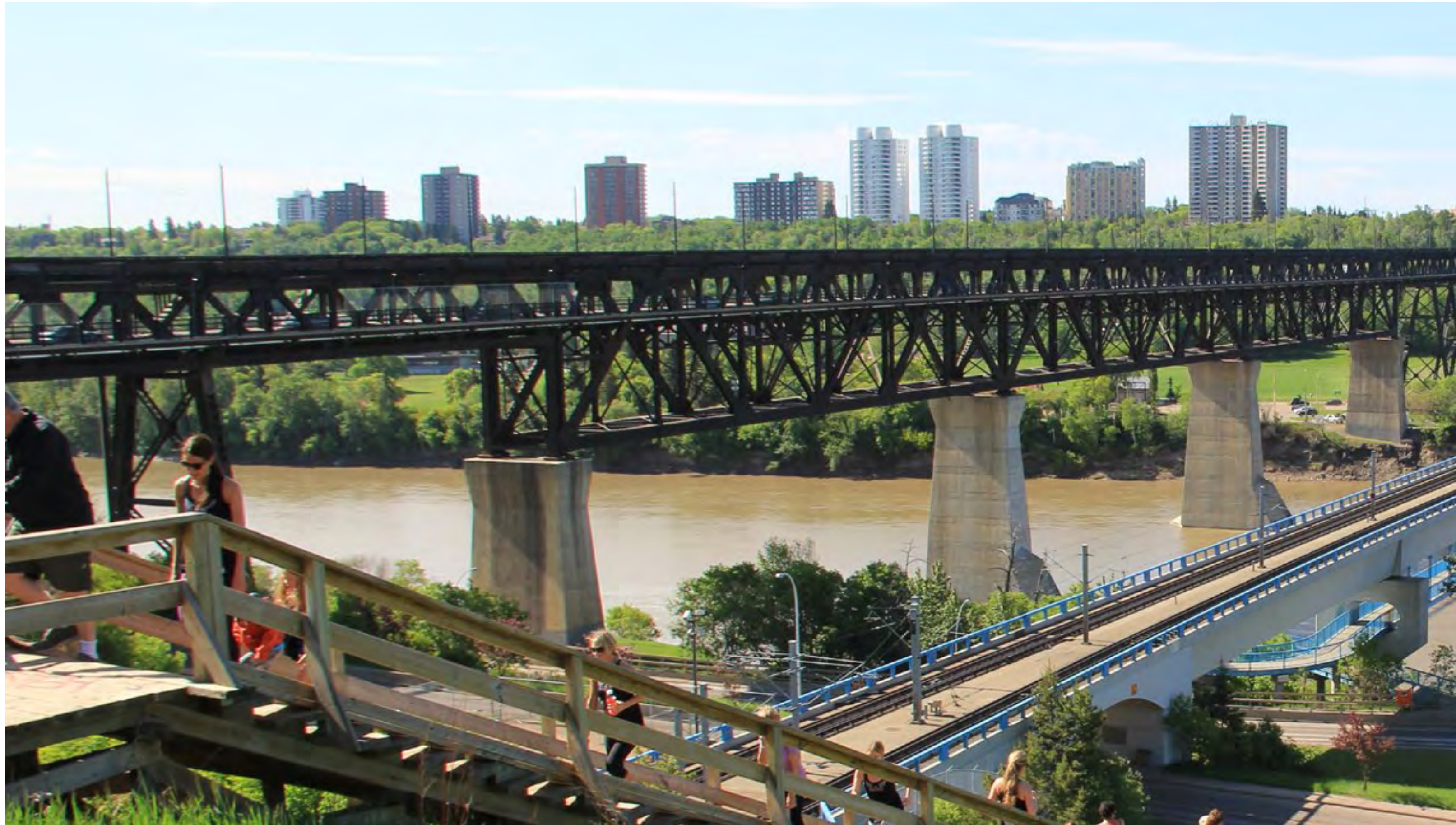
View from Ezio Faraone Park at top of existing stairs to High Level Bridge
