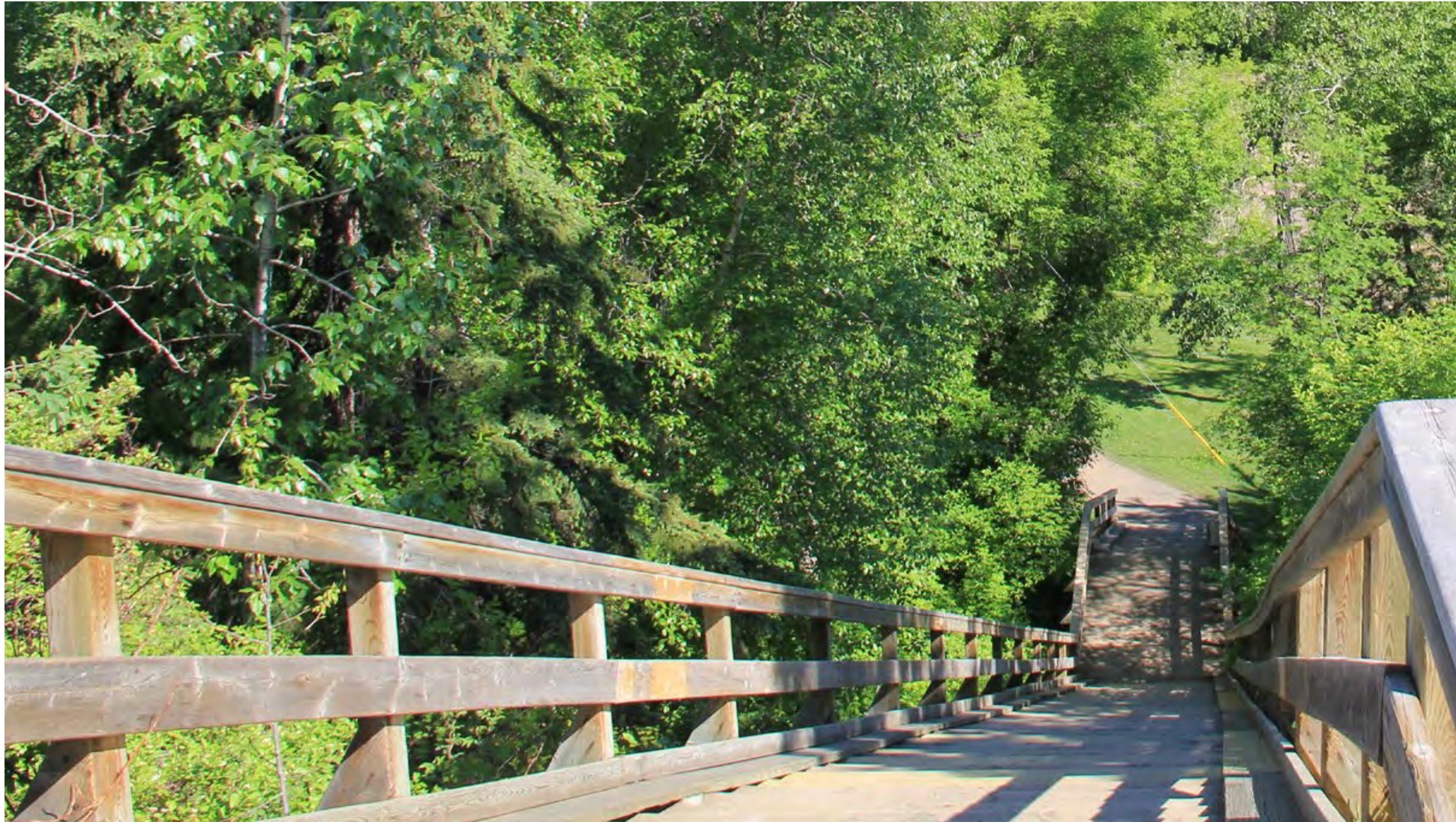
View down existing stairs at 105 Street and Saskatchewan Drive
