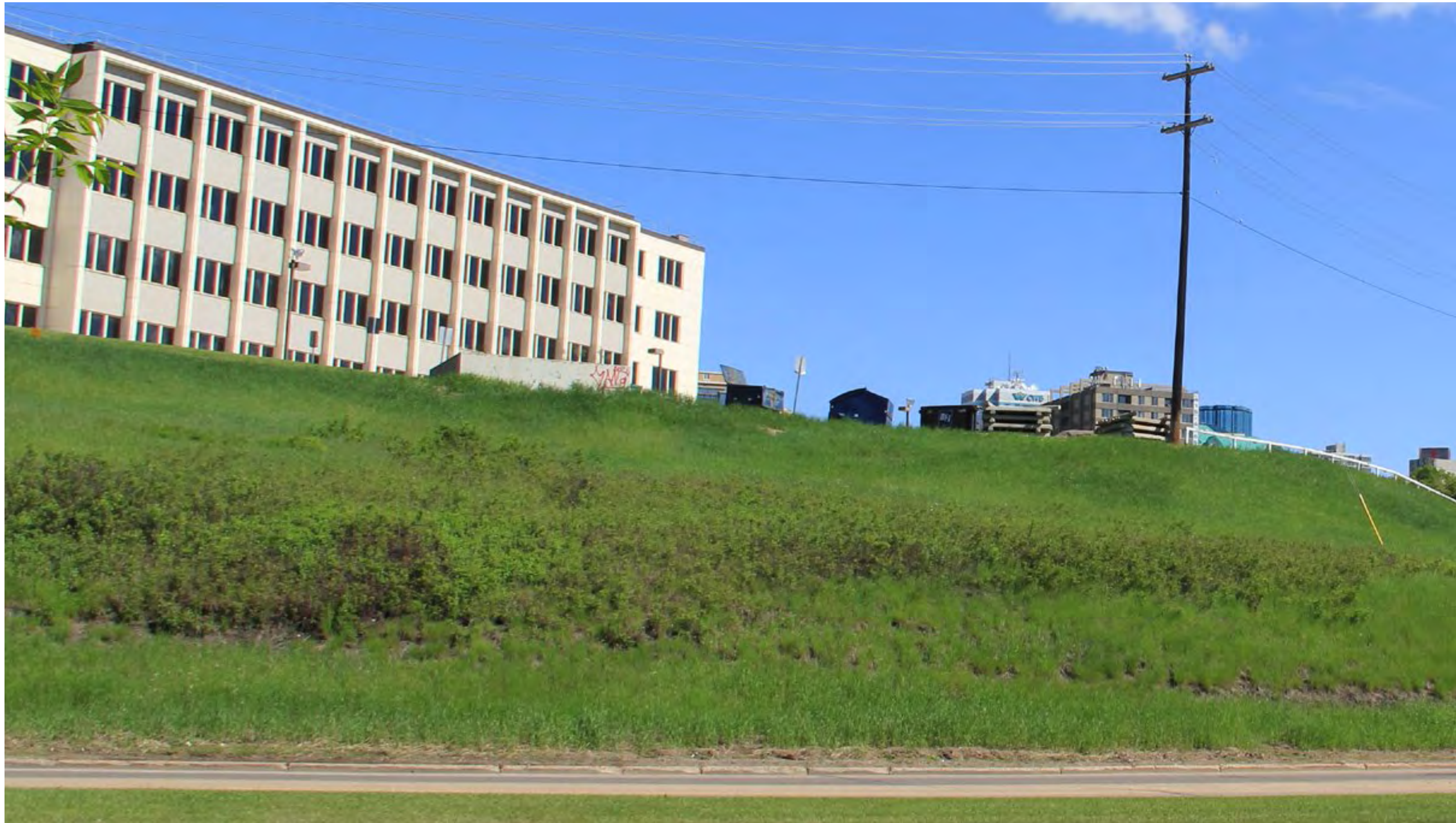
View across River Valley Road to existing slope at 106 Street alignment
