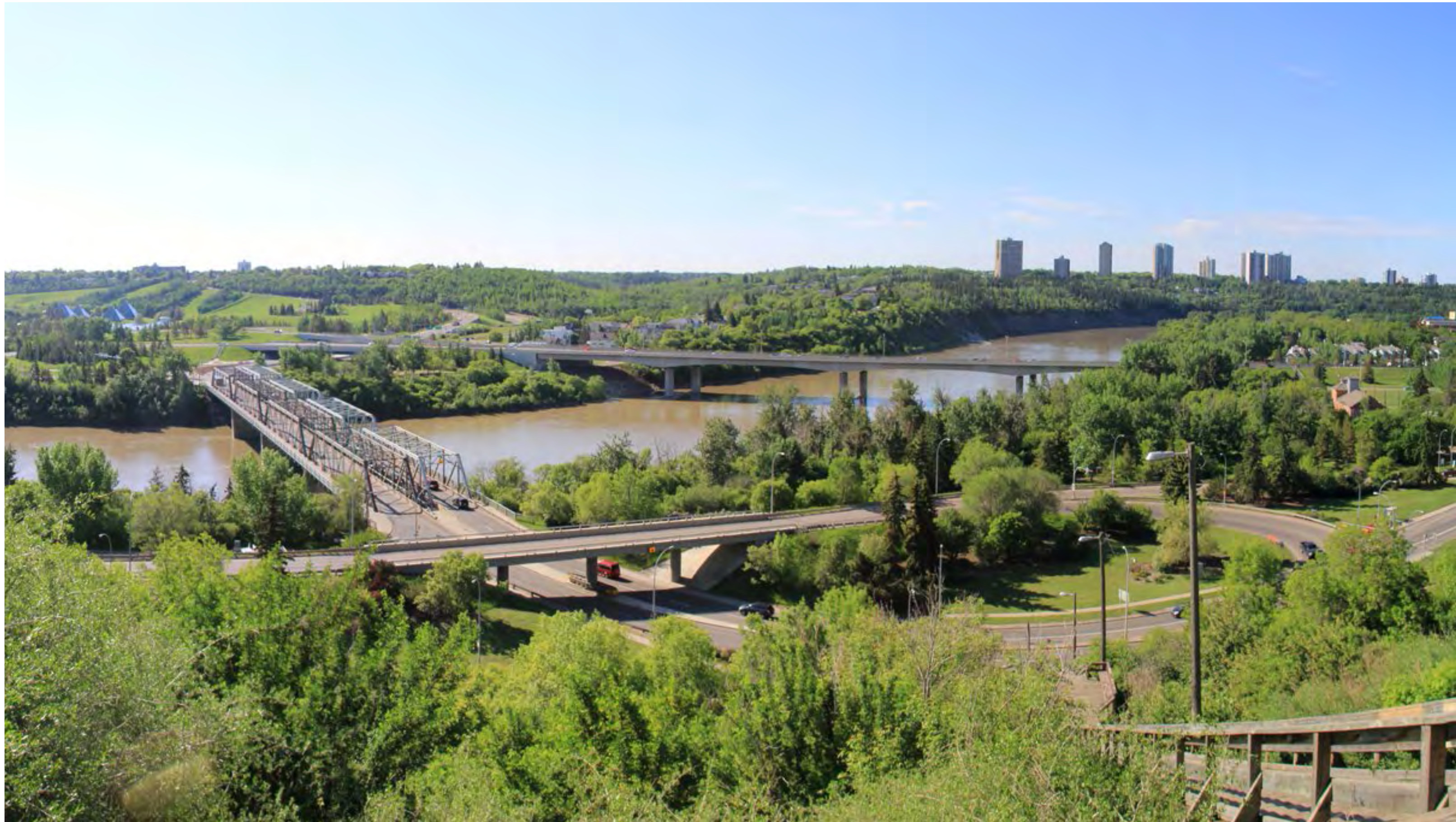
View of the top of the existing stairs at 100 Street and McDougall Hill
