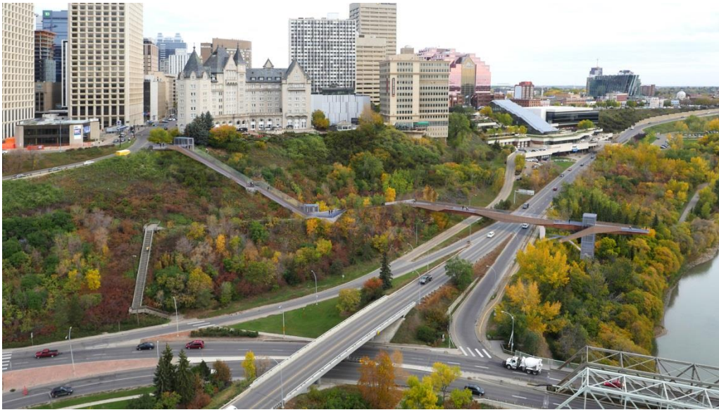
Plate 1.1. Proposed RVMA project locations and components (DIALOG 2015a). Note that the image does not depict the retained lower portion of existing wooden stair and the trail connector between the stair and promenade.
