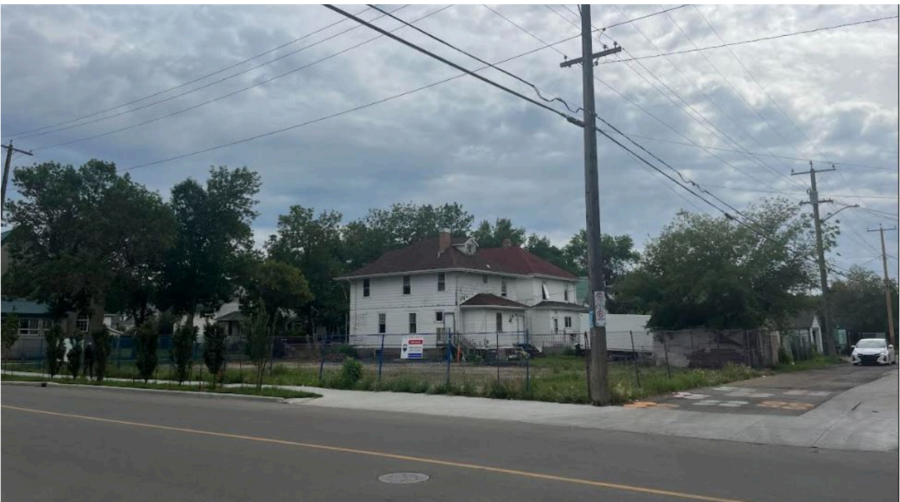
View of the site looking southeast from 115 Avenue NW
