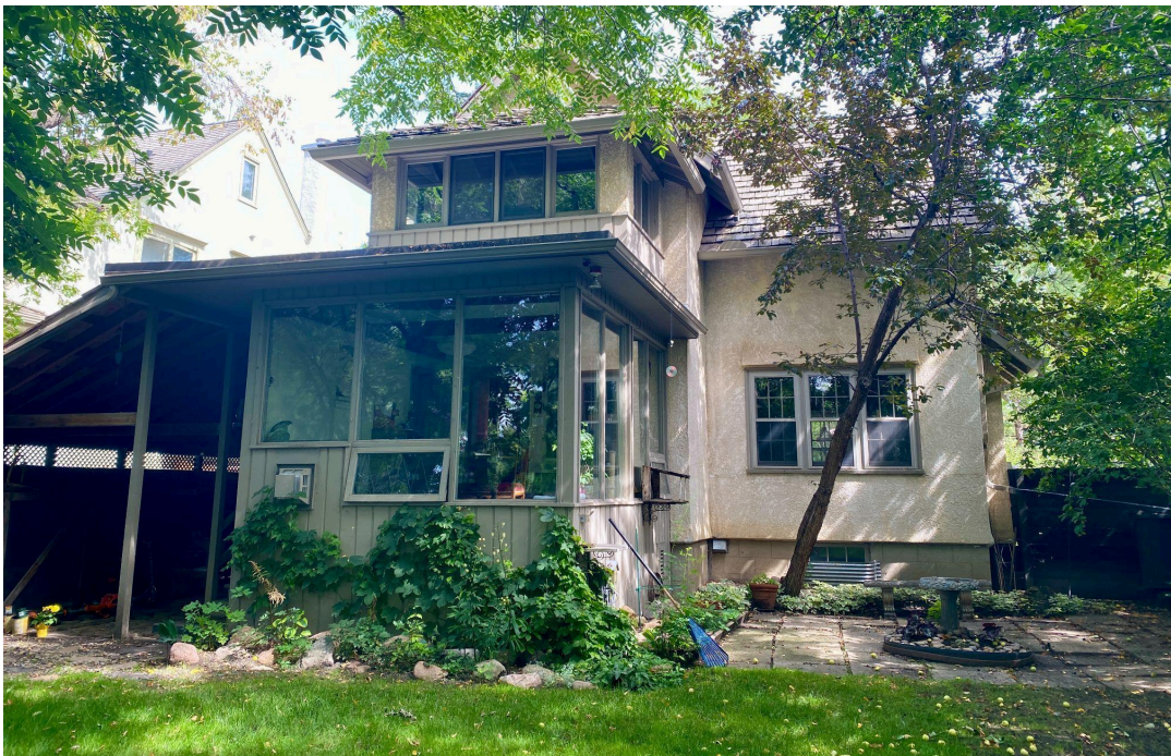
View of west (rear) elevation, looking east
