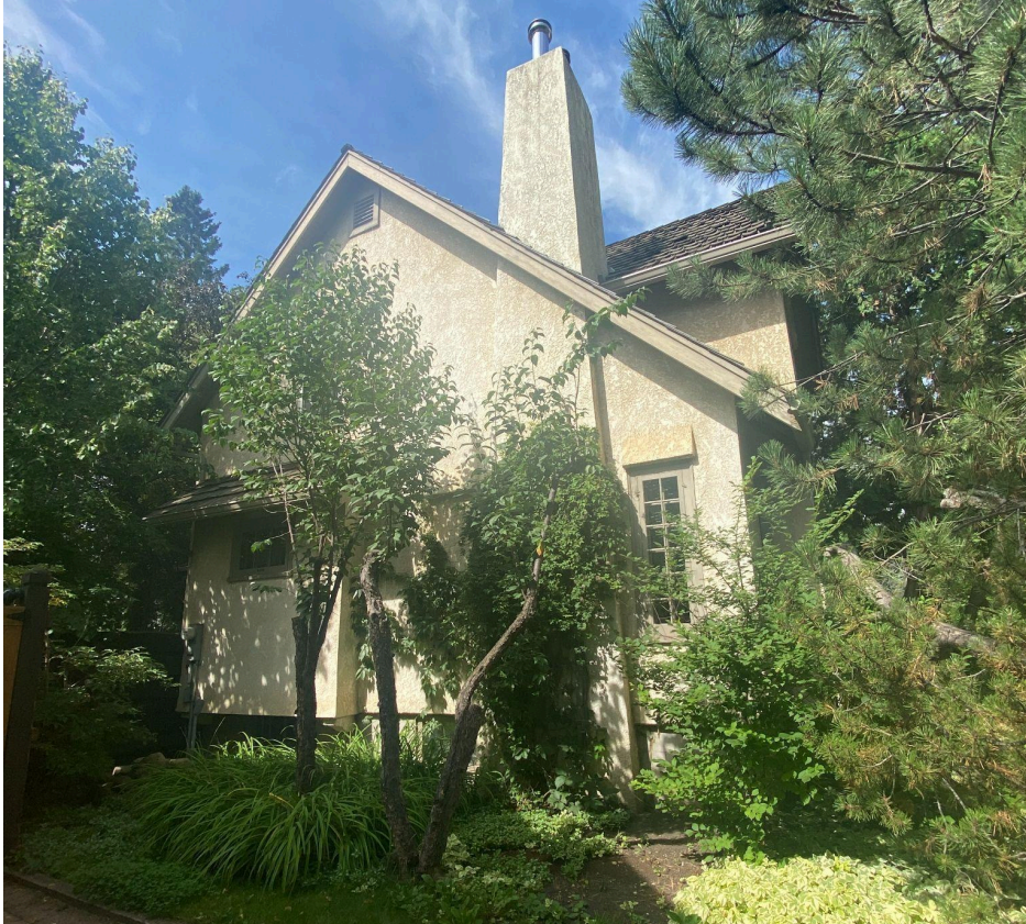
View of south (side) elevation, looking north.
