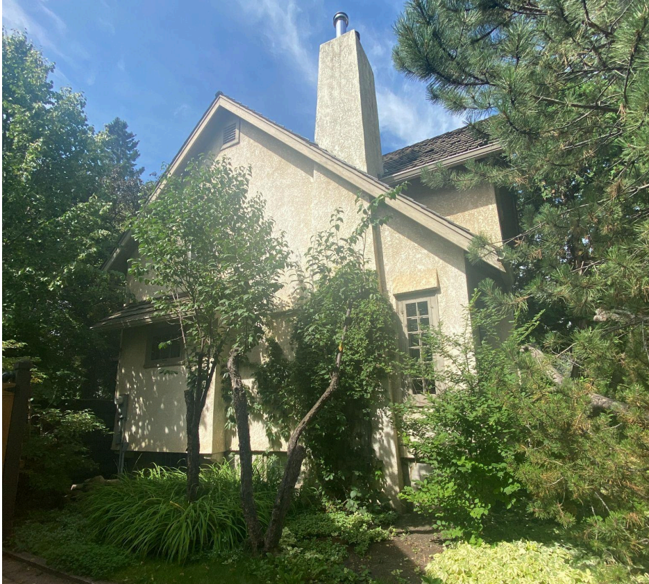
View of south (side) elevation, looking north.
