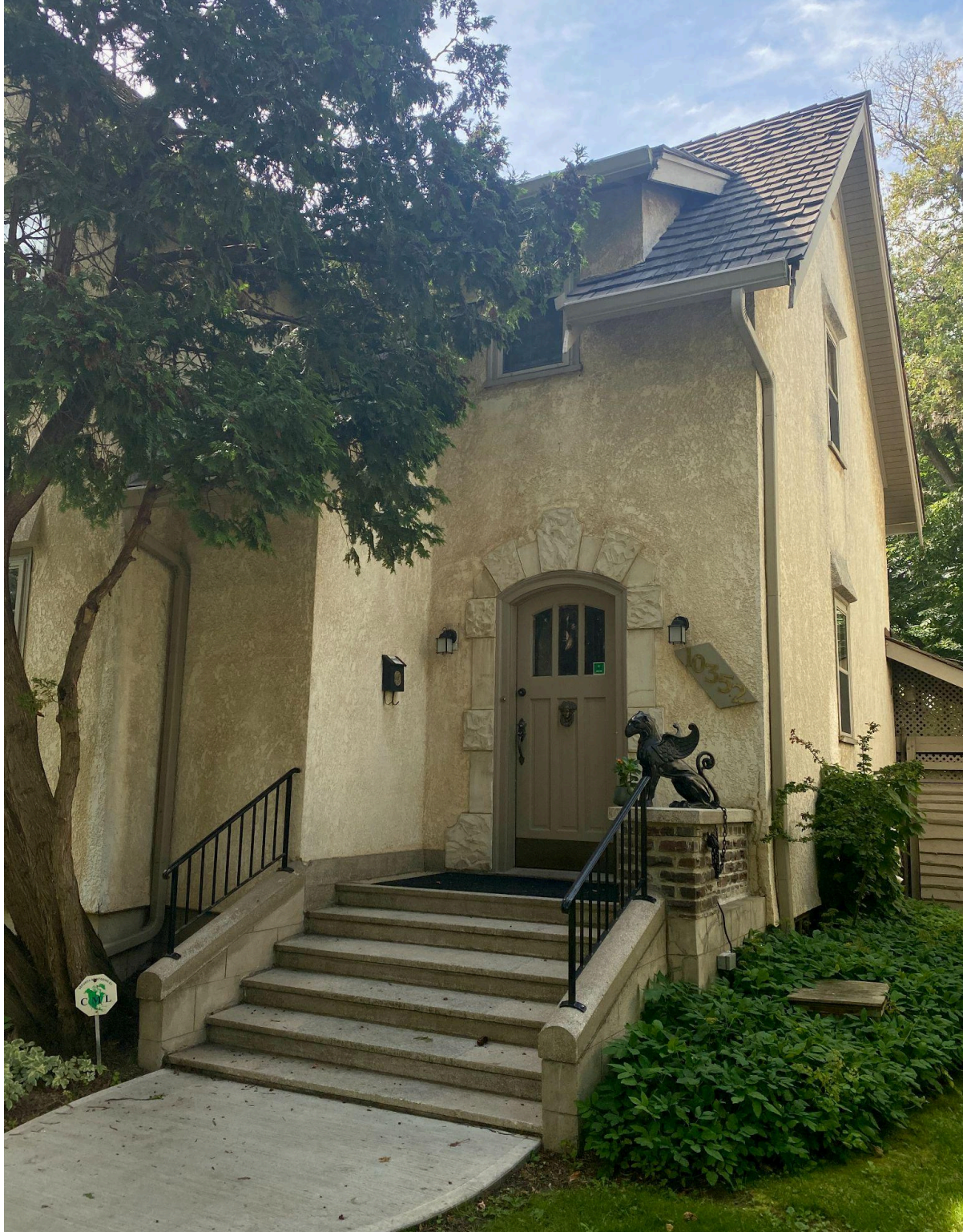
View of northeast (side and front) elevation, looking south
