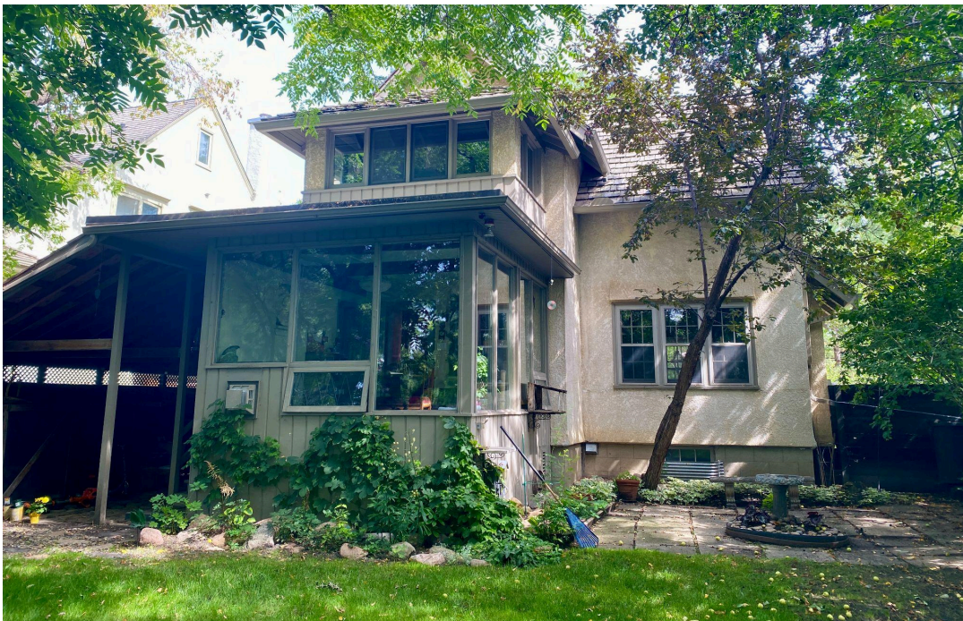
View of west (rear) elevation, looking east
