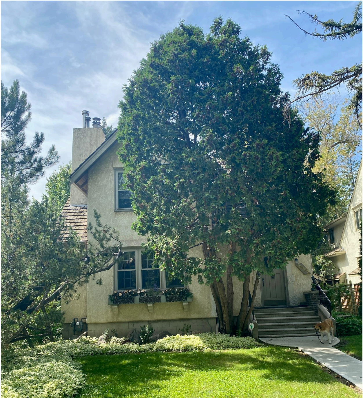
View of east (front) elevation, looking west from 127 Street NW
