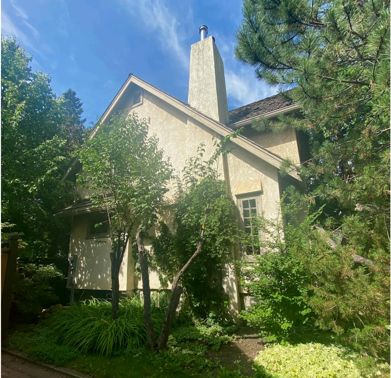
View of south (side) elevation, looking north
