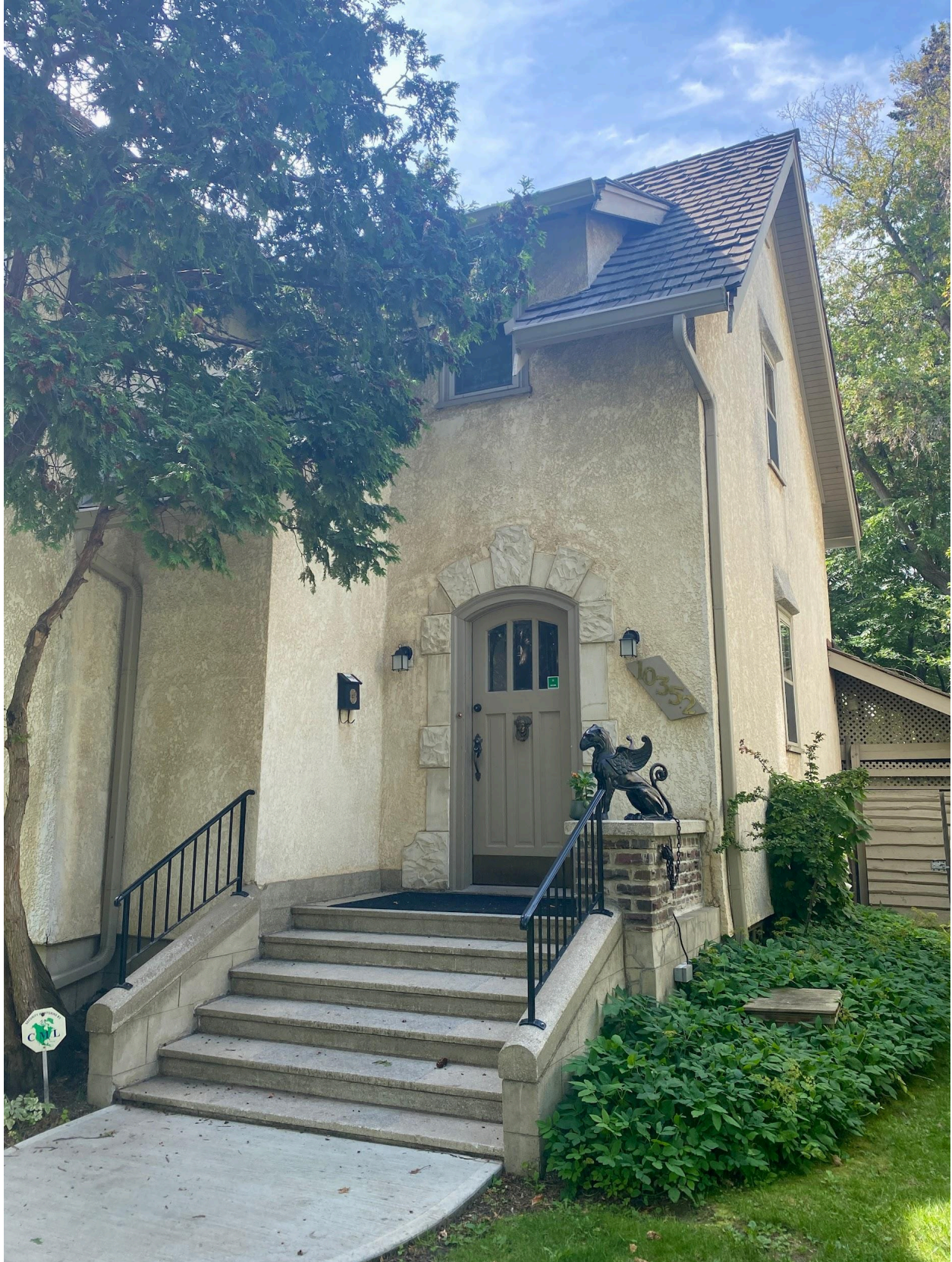
Front entrance and north (side) elevation
