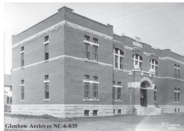
IMAGE CONNAUGHT ARMOURY, SOUTH EDMONTON, EDMONTON, ALBERTA, 1914, (CU154042) SOURCE MCDERMID STUDIO. COURTESY OF COLLECTION, LIBRARIES AND CULTURAL RESOURCES DIGITAL COLLECTIONS, UNIVERSITY OF CALGARY.
