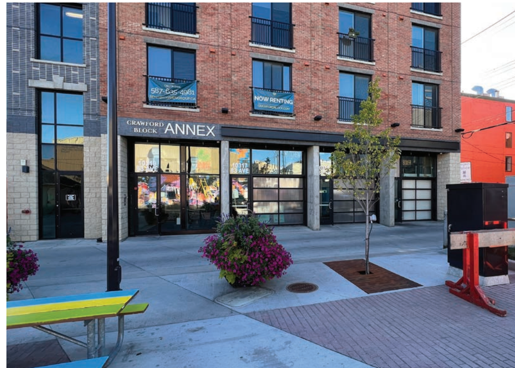
IMAGE STRATHCONA BACK STREET ENTRANCE
