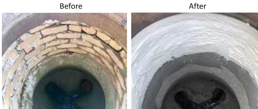
Figure 4.1-1: Typical Manhole Before and After Sealing
