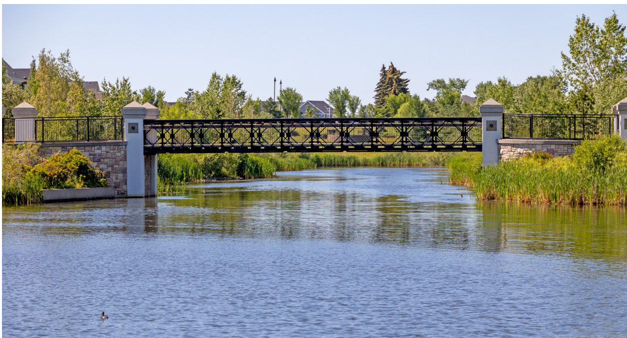
The Griesbach Stormwater Management Facility
