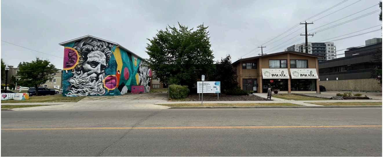
View of site looking north across 105 Avenue NW
