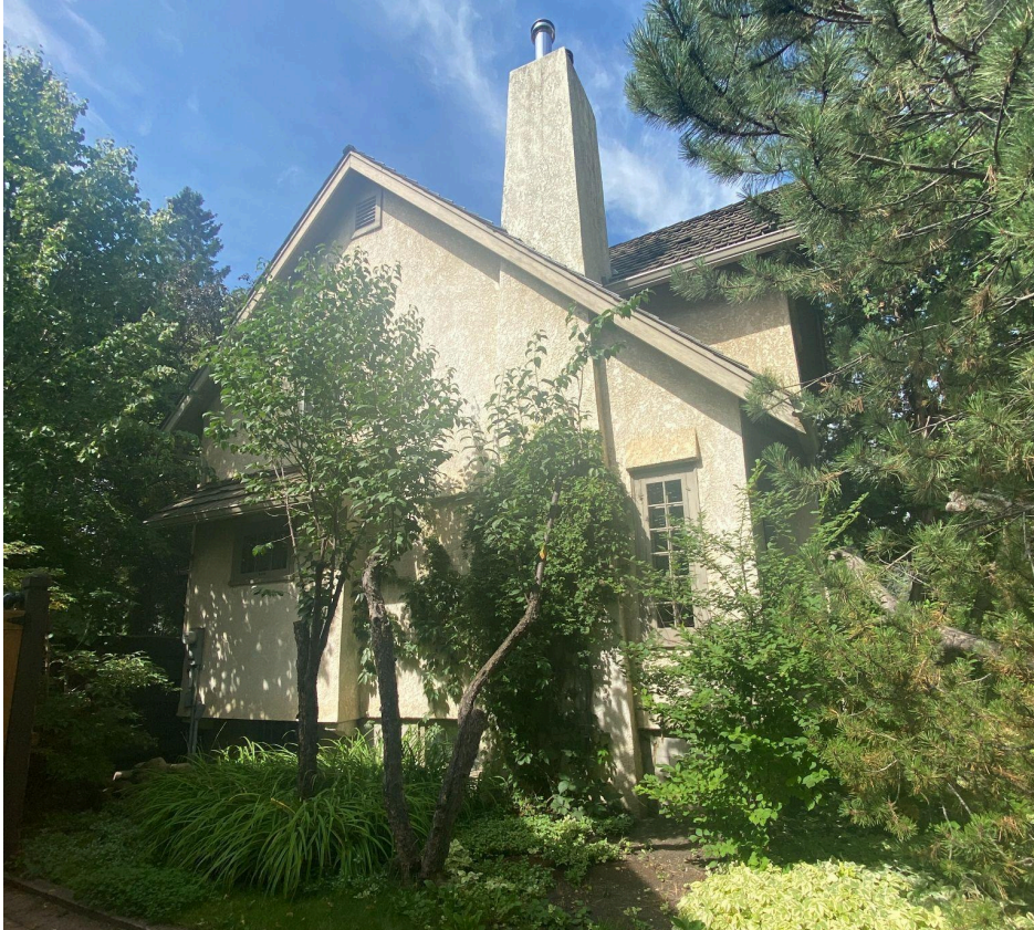
View of south (side) elevation, looking north.
