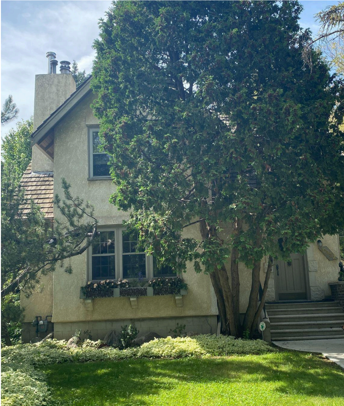
View of east (front) elevation, looking west from 127 Street NW
