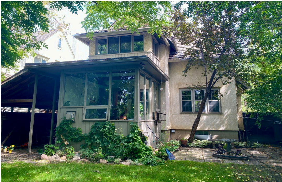
View of west (rear) elevation, looking east
