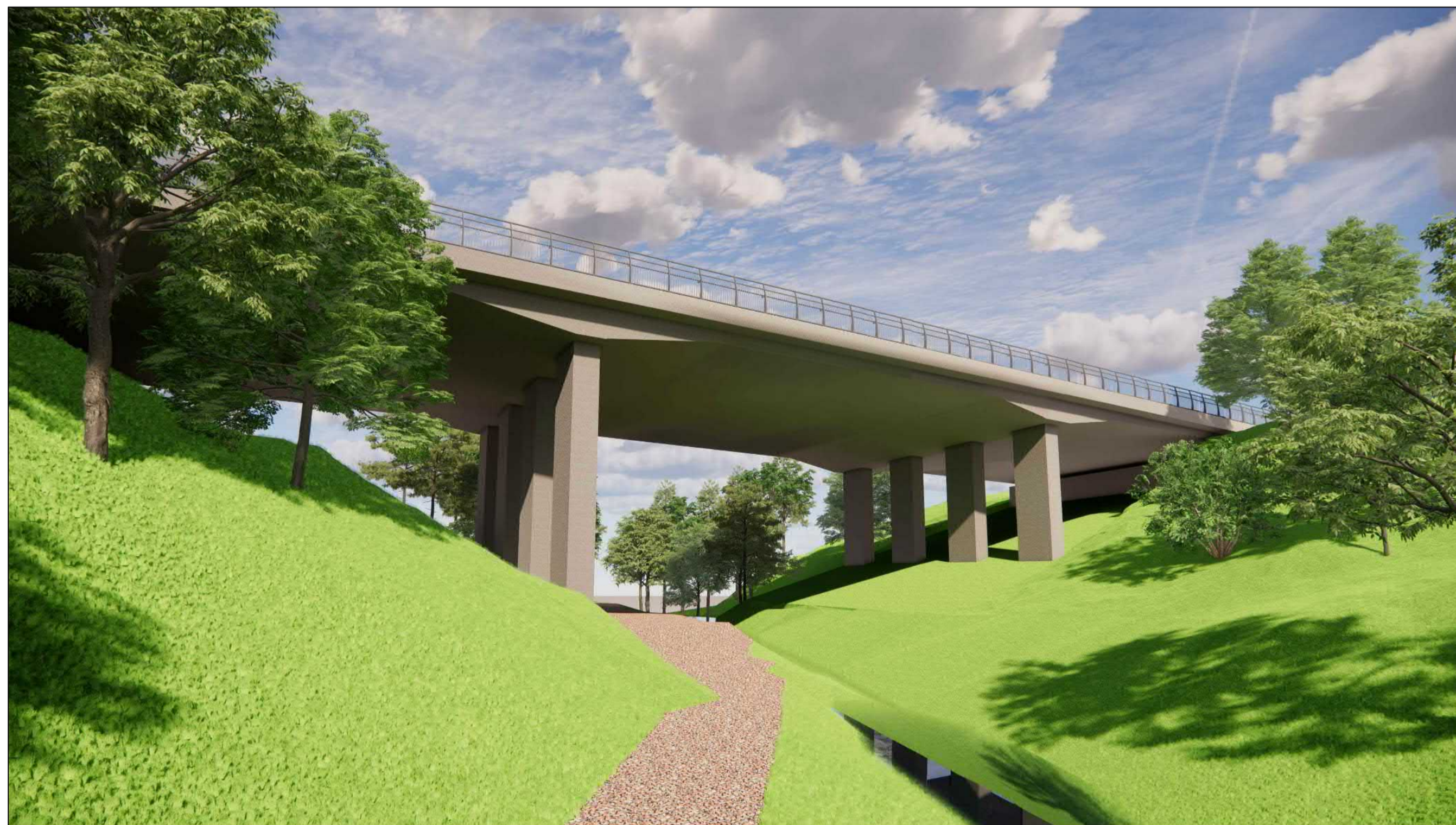
PHOTO THREE SPAN HAUNCHED CONCRETE GIRDER OPTION
