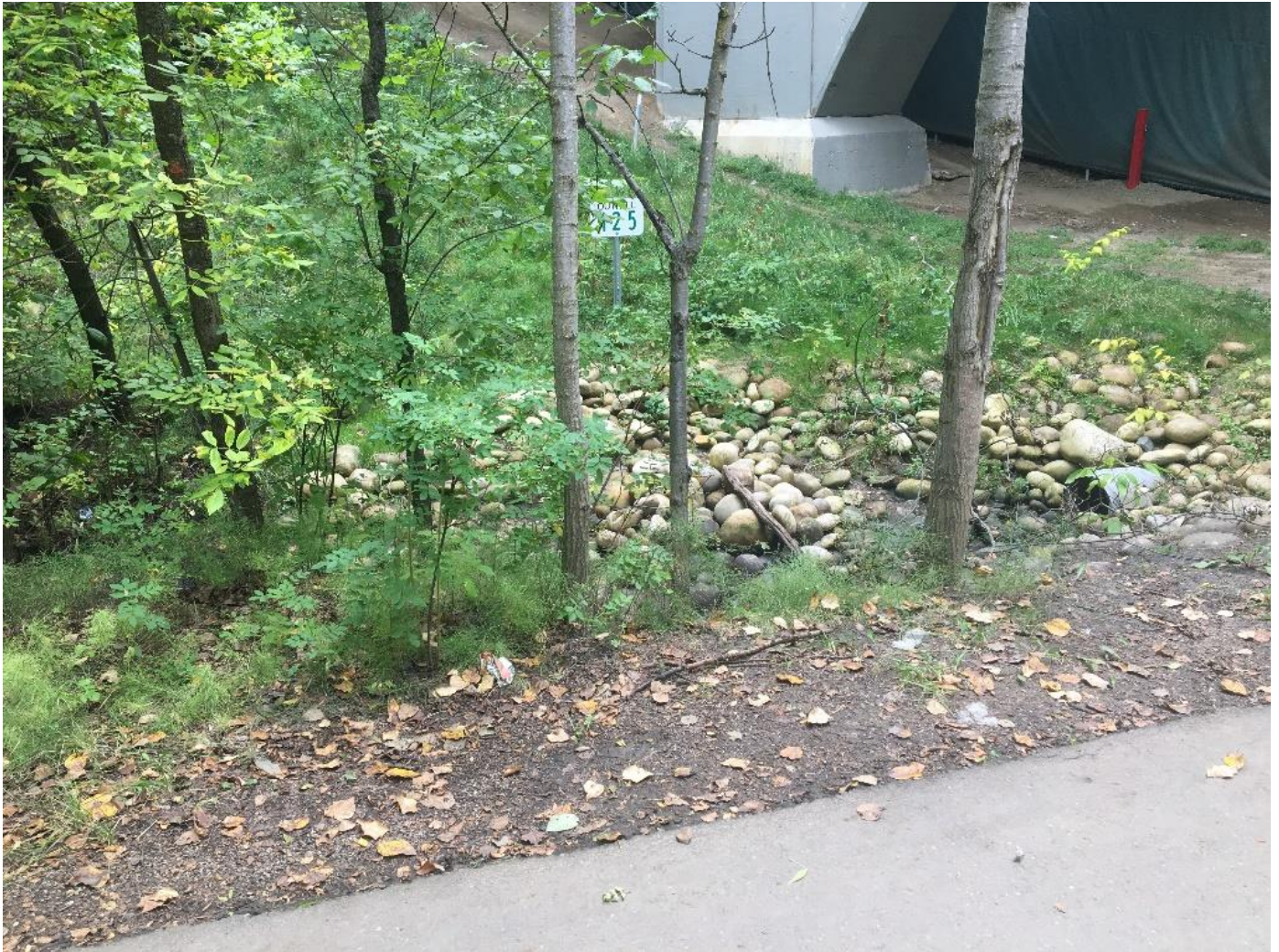
Figure 3-3 Outfall 125 in Unnamed Watercourse
