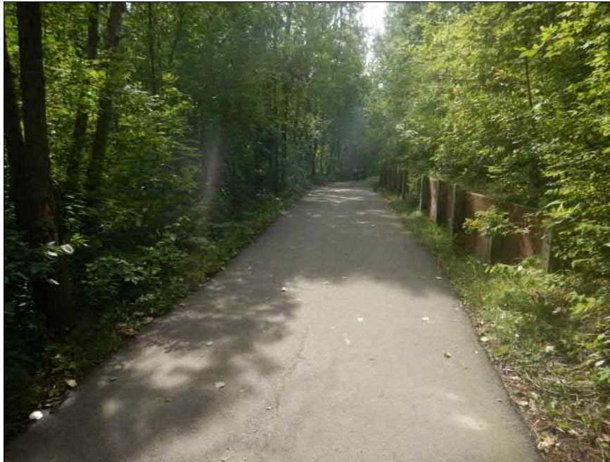
PHOTO 2 TIMBER RETAINING WALL ALONG WEST SIDE OF MULT-USE TRAIL TOWARDS SOUTH
