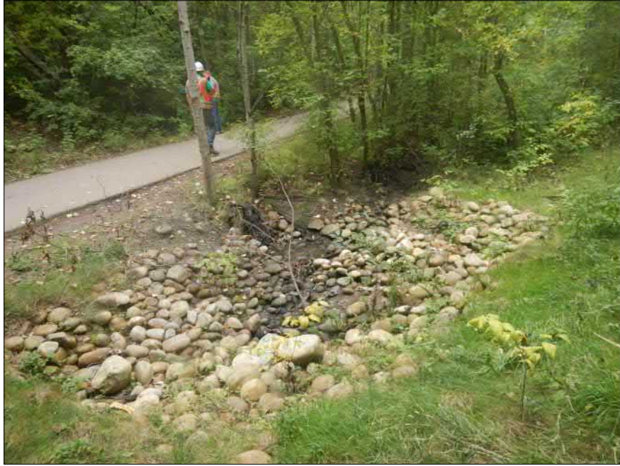
PHOTO 5 OUTFALL ON EAST SIDE OF MULTI-USE TRAIL FROM CHURCHILL CRESCENT
