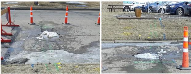
Figure 3.0-1 Active Subsidence around a Failed MH
