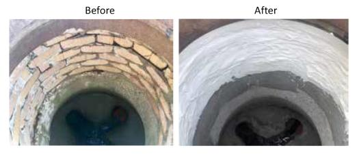
Figure 4.1-1: Typical Manhole Before and After Sealing
