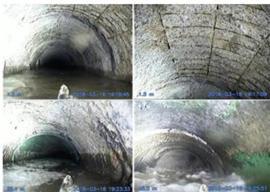
Figure 3.0-1 Deterioration of Small Trunks
