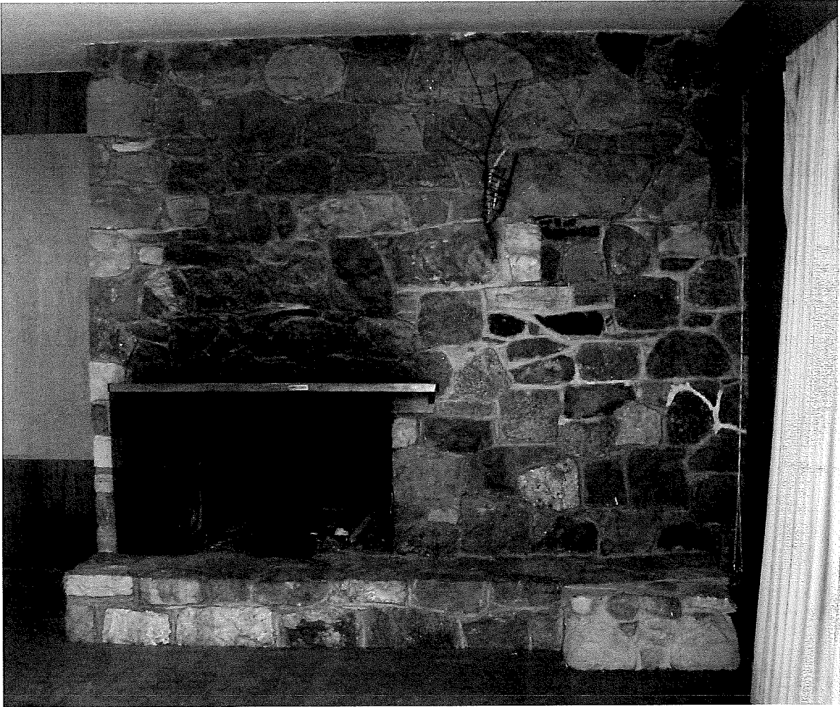
Cut Fieldstone Fireplace (ground level)
