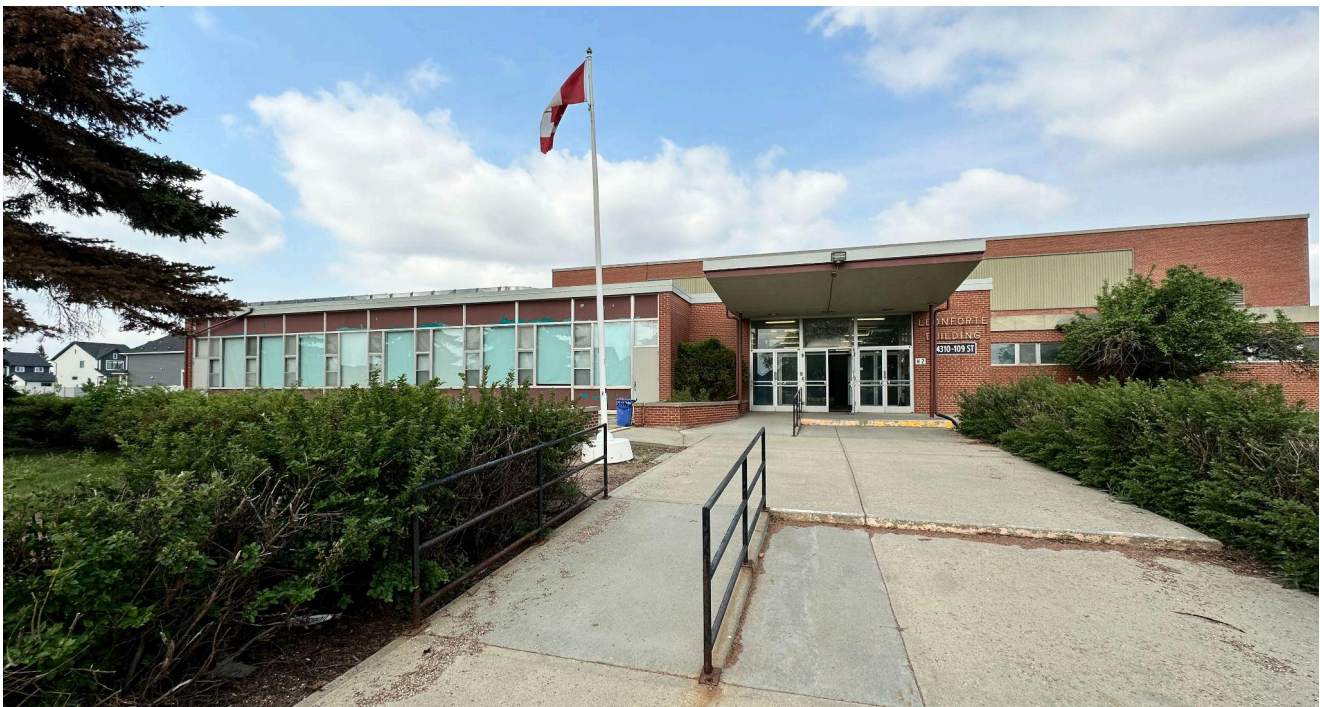
View of the main entrance (looking west).
