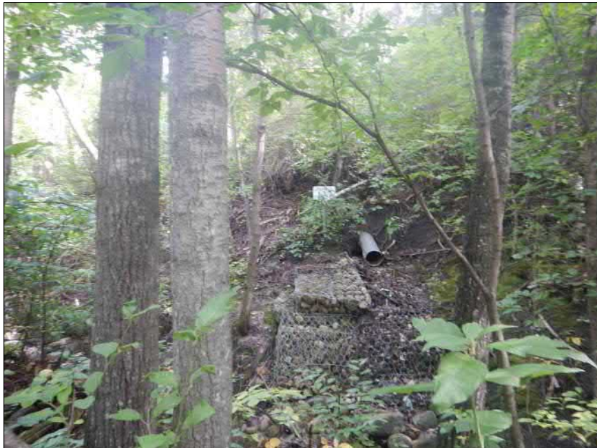
PHOTO 12 OUTFALL ON EAST RAVINE SLOPE SOUTH OF BRIDGE
