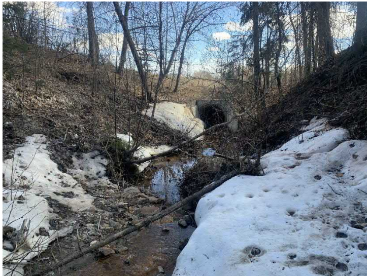
Photograph 2 Downstream showing channel and outfall structure at Transect T1.
