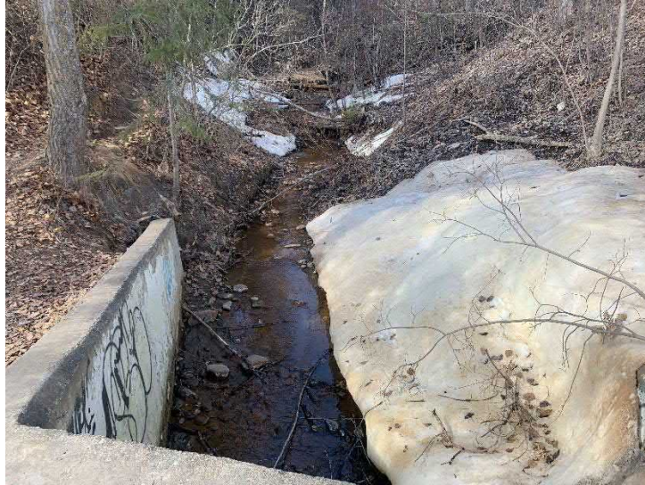
Photograph 1 Upstream showing channel at Transect T1.
