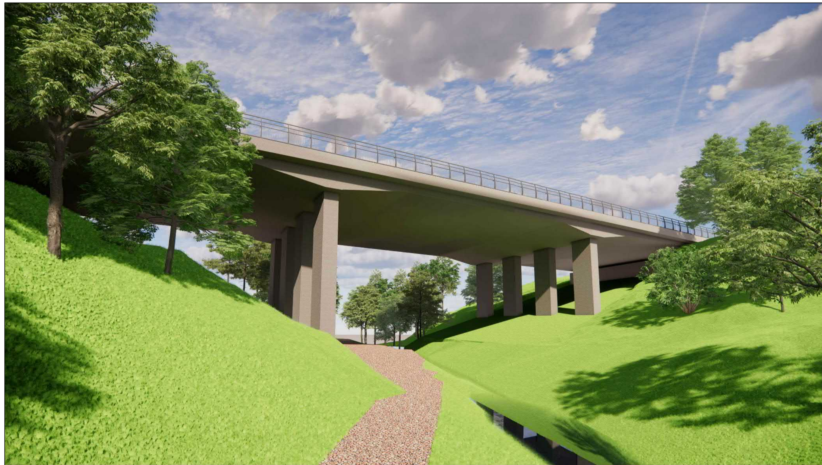
PHOTO THREE SPAN HAUNCHED CONCRETE GIRDER OPTION
