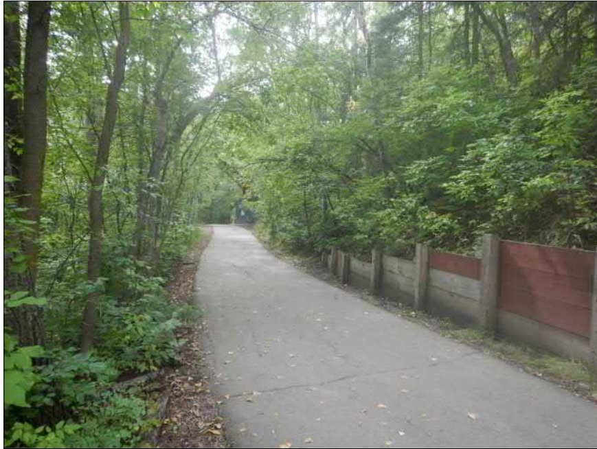
PHOTO 3 SOUTH END OF TIMBER RETAINING WALL NORTH OF BRIDGE
