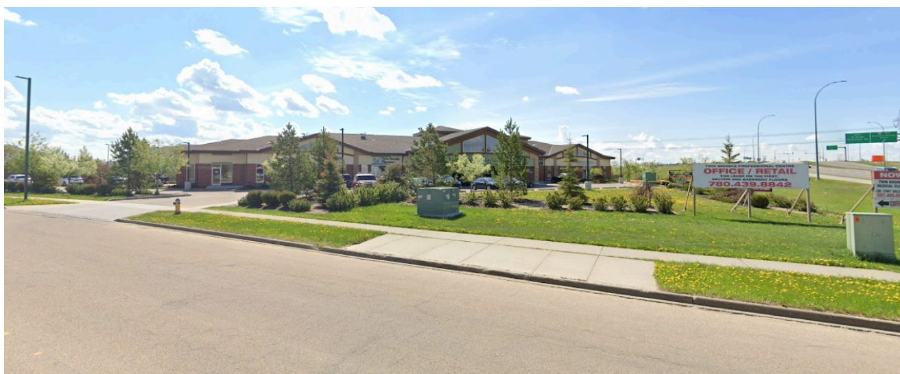
View of the site looking southeast from 9 Avenue NW
