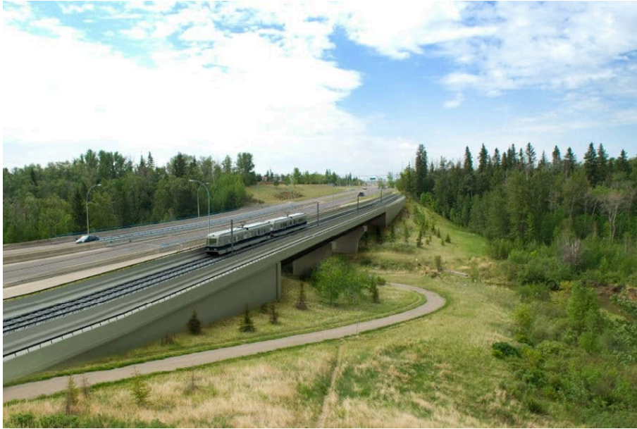
Figure 1: Project area showing proposed LRT bridge across Blackmud Creek, looking South
