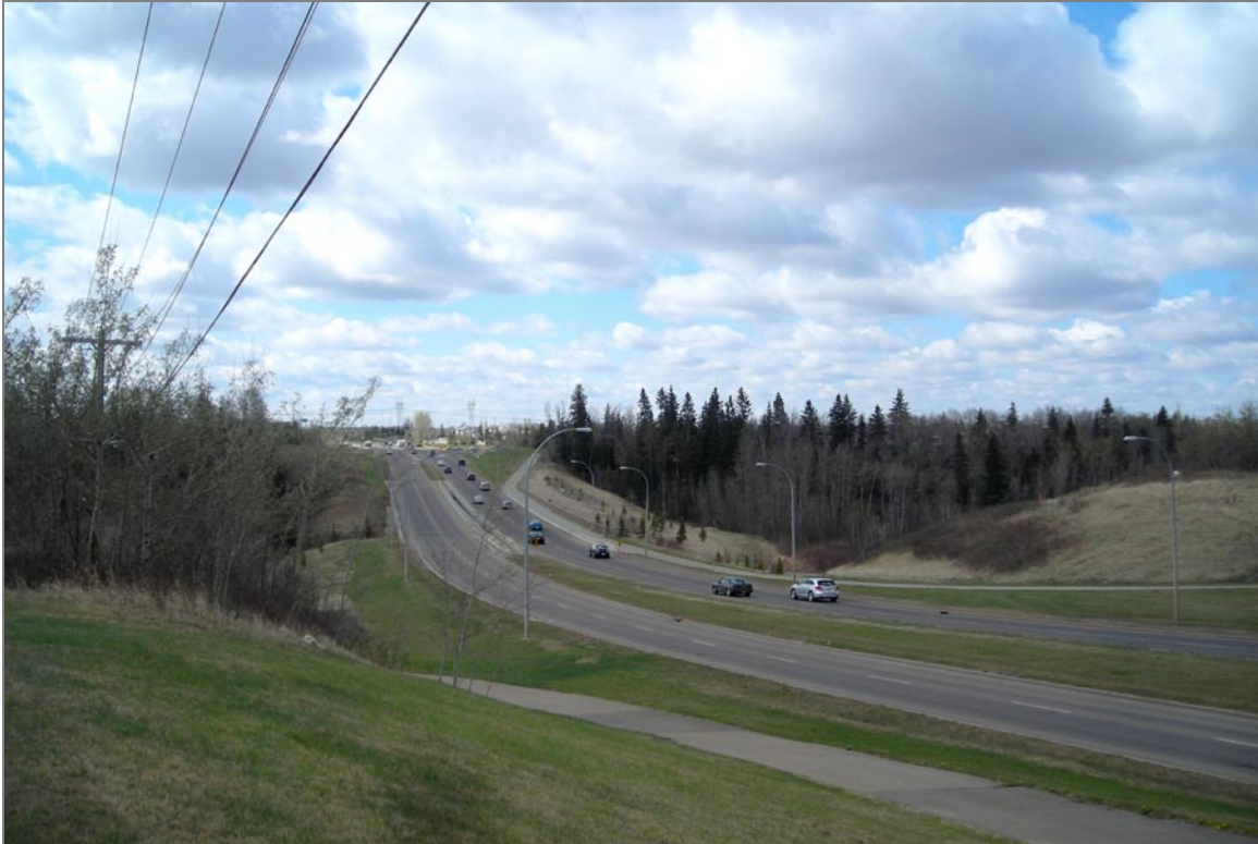
Photo 1: View southeast of current landscaping and roadway disturbances at the proposed Blackmud Creek Crossing
