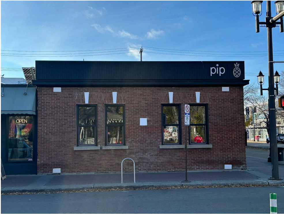
View of front (north) elevation, looking south from 83 Avenue NW.
