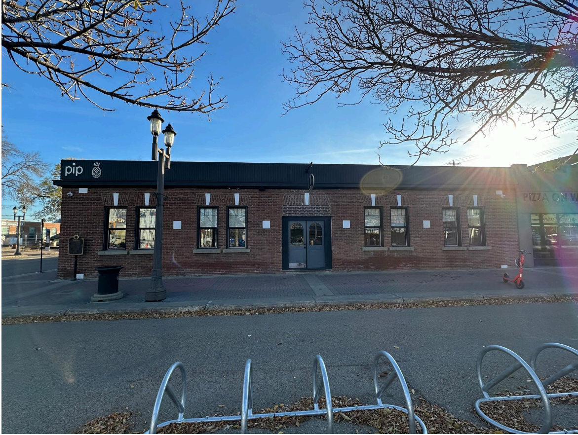
View of side (west) elevation, looking east from Calgary Trail NW.
