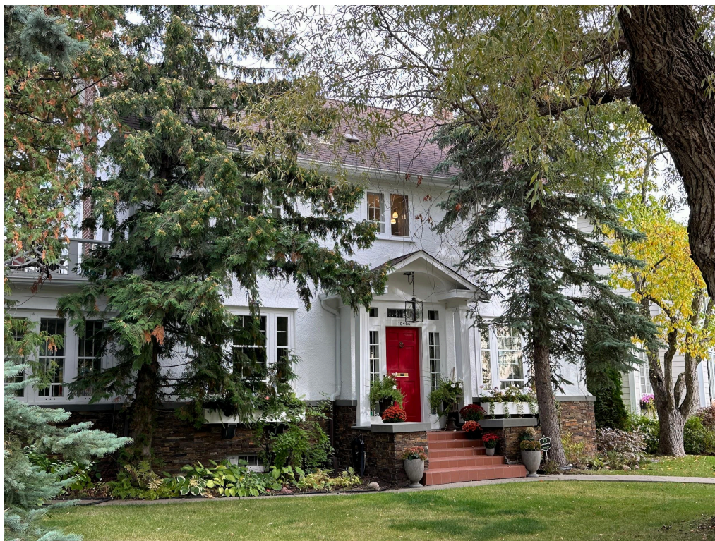
View of front (south) and side (west) elevations, looking northeast from Connaught Drive NW.
