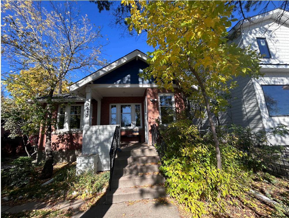
View of front (south) elevation, looking north from 103 Avenue NW.
