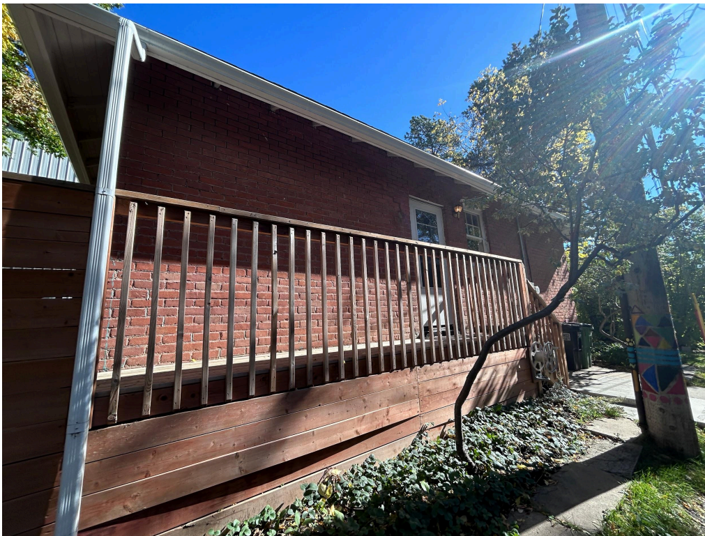
View of side (west) elevation, looking southeast from adjacent lane.
