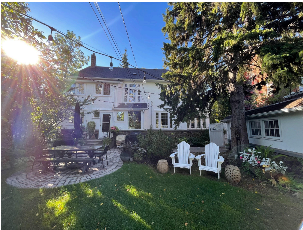
View of rear (north) elevation, looking south from property rear yard.
