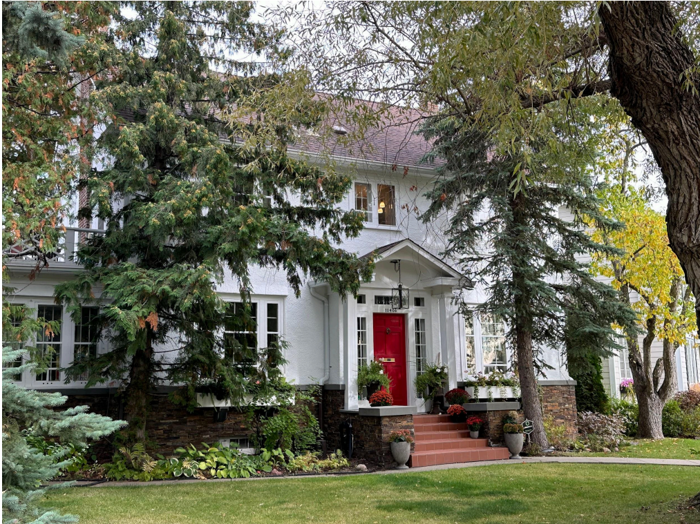
View of front (south) and side (west) elevations, looking northeast from Connaught Drive NW.
