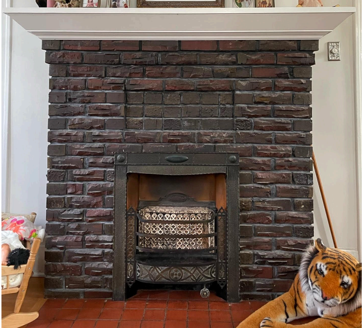
View of clinker brick fireplace.
