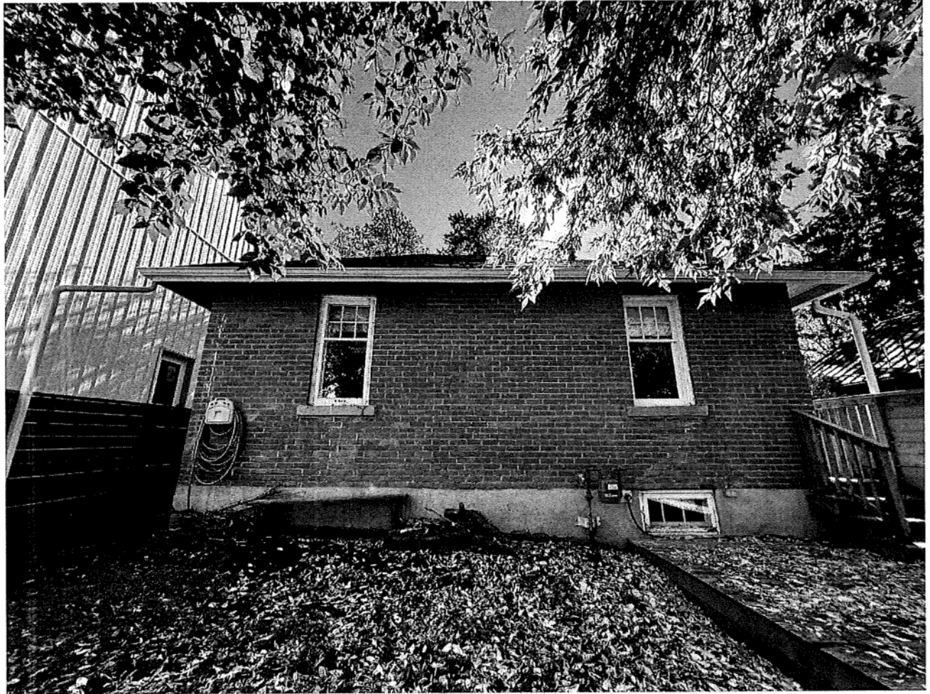
View of rear (north) elevation, looking south from property rear yard.
