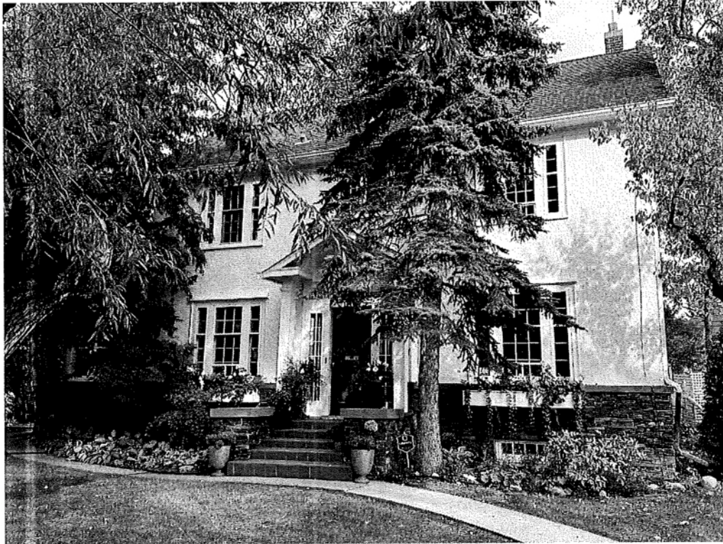
View of front (south) elevation, looking northwest from Connaught Drive NW.
