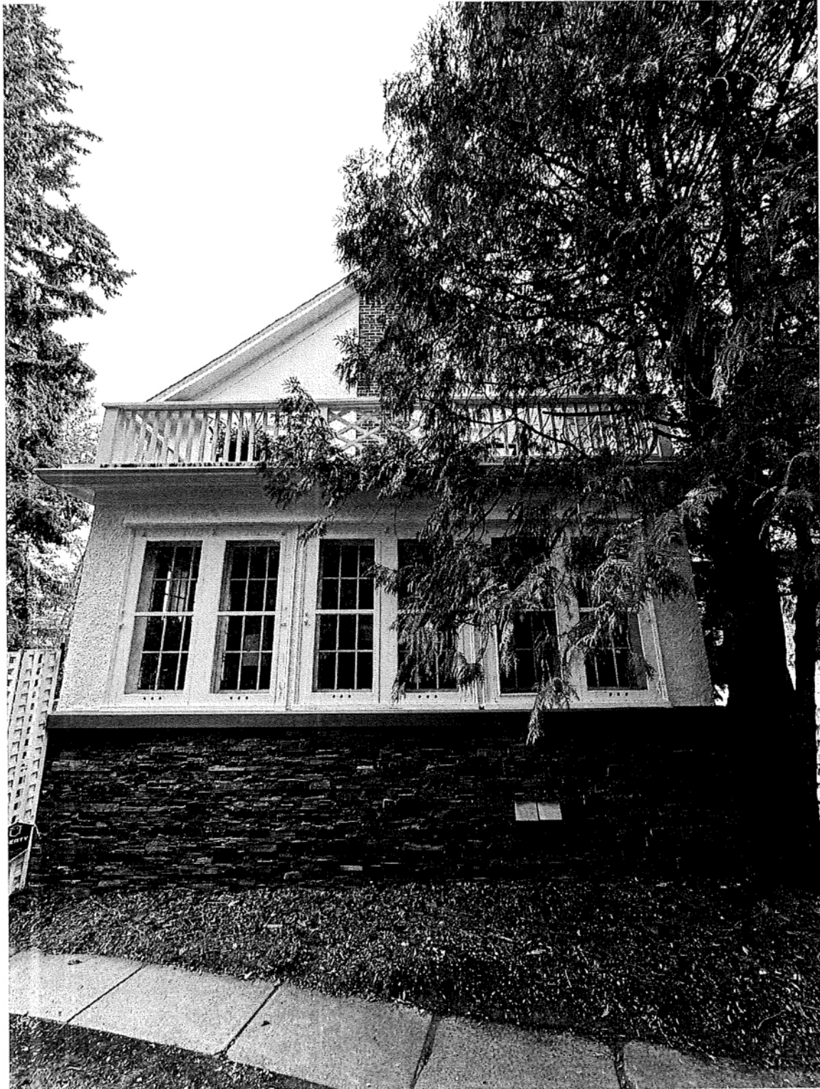
View of side (west) elevation, looking east from property side yard.
