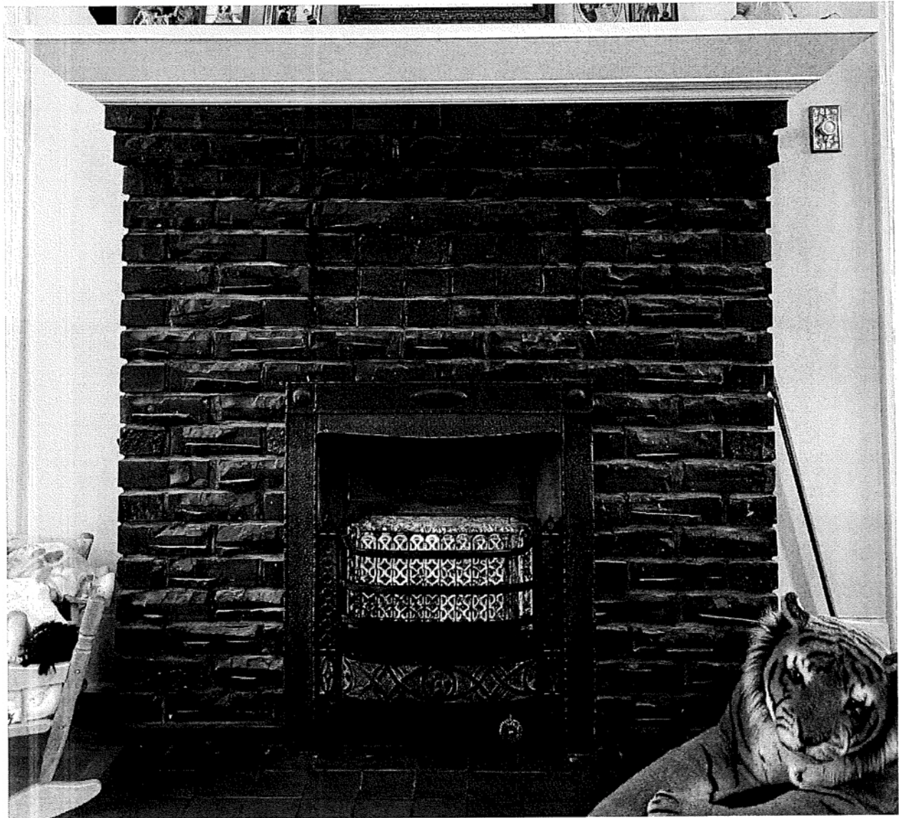
View of clinker brick fireplace.
