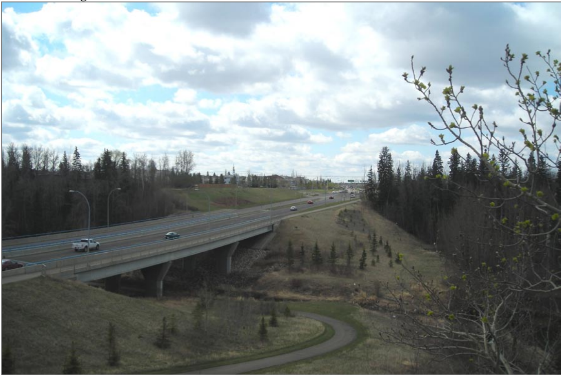
Photo 2: View southeast of current roadway and bridge disturbances on the west side of the bridge at the proposed Blackmud Creek crossing.
