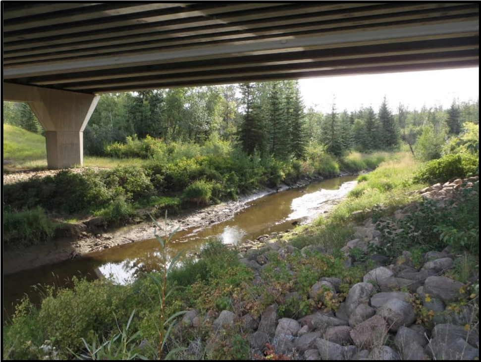
Photo 1 Blackmud Creek facing east under existing bridges
