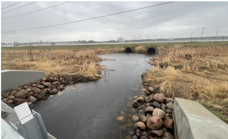
Photo plate #23: View towards highway 15 culverts (May 16,2024).
