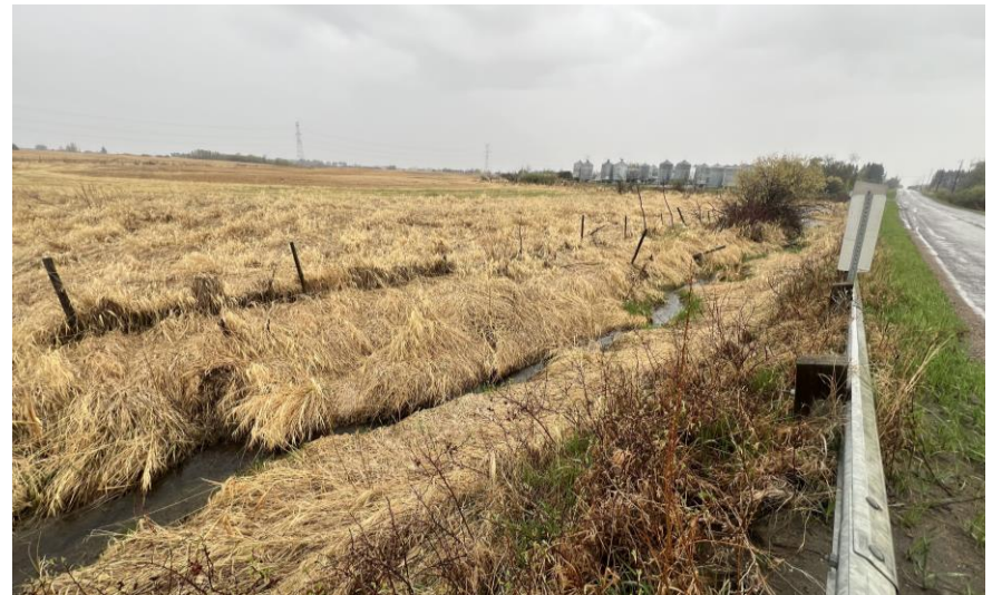
Photo plate #16: Showing upstream from bridge, showing channel constraint between field and 18 Street (May 16, 2024).
