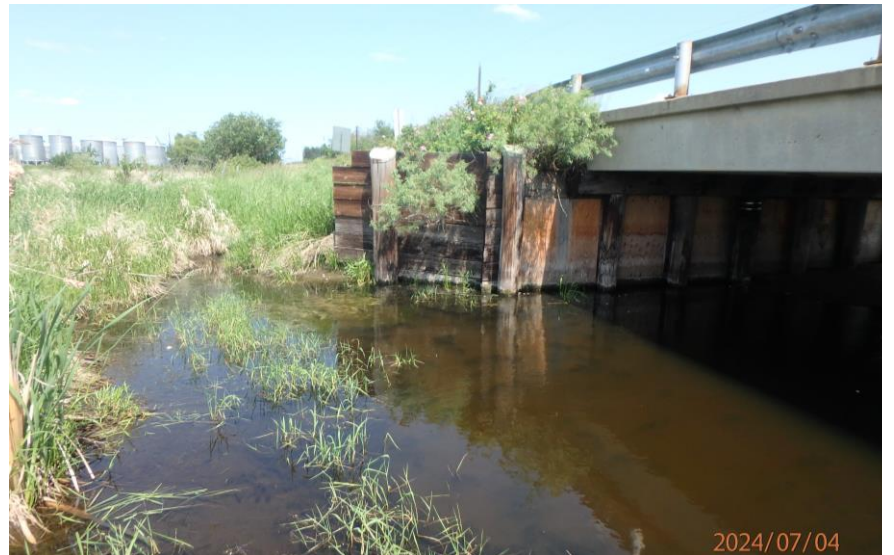
Photo plate #28: View of upstream side of bridge (July 4,2024.)
